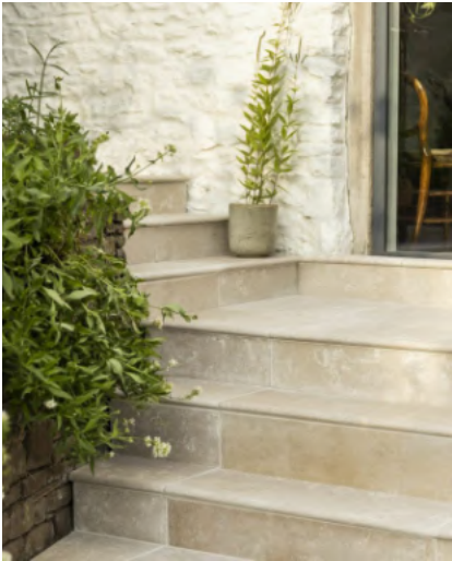
1 Stepped access from building entrance
