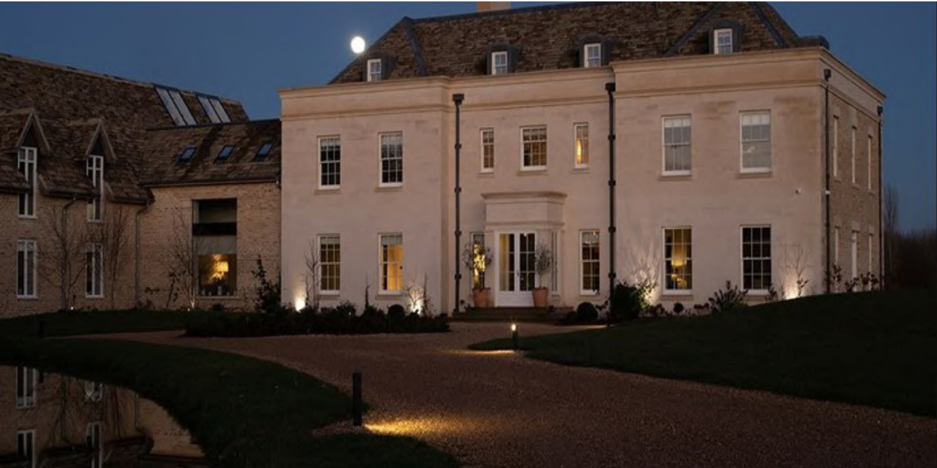
Lighting to highlight building entrances
