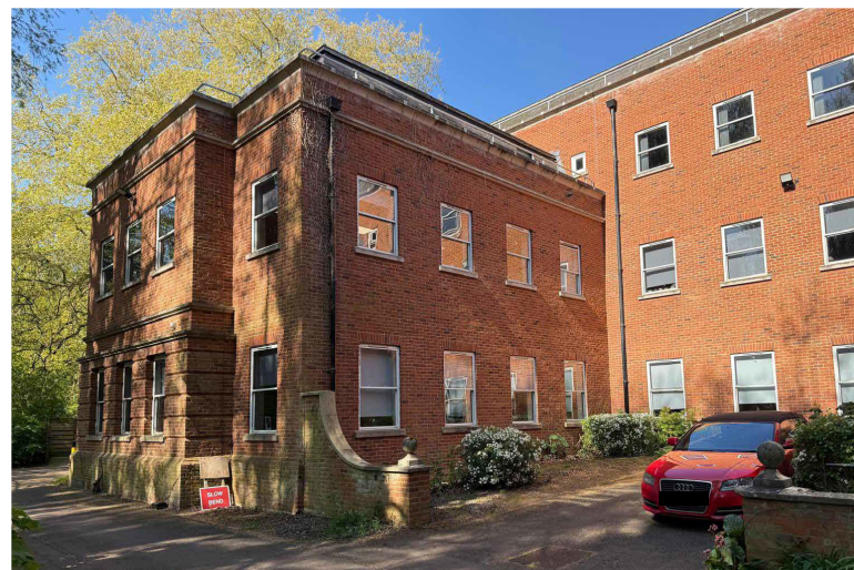
5 South east courtyard
