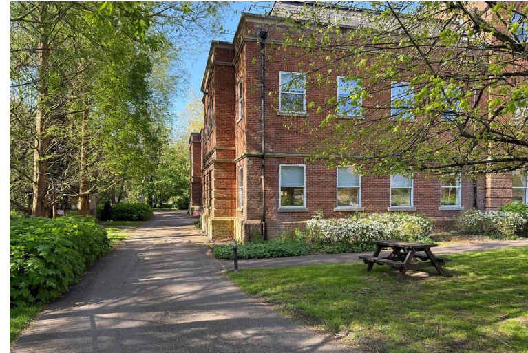
3 North east elevation, main building frontage
