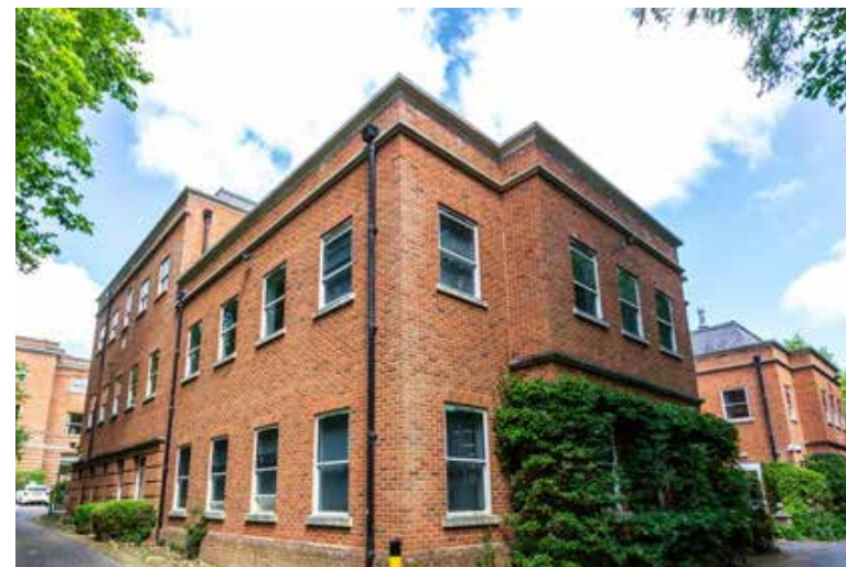
6 South east / west corner
