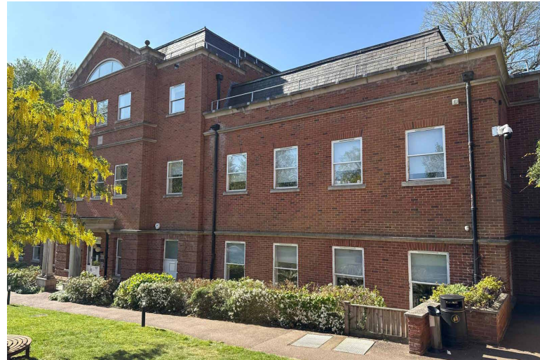
2 North east elevation, main building frontage
