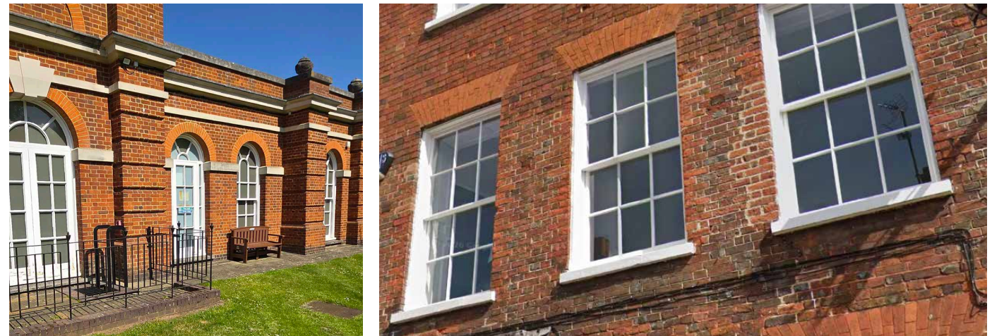
FIGURE 16: EXISTING WINDOWS WITH WINDOW BARS AT THE PRIORY AND IN LOCAL AREA
