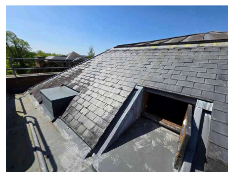
FIGURE 11: ROOF DOOR RECESS
