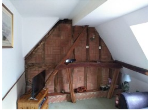
Figure 6 - Original timbers to existing residential accommodation
