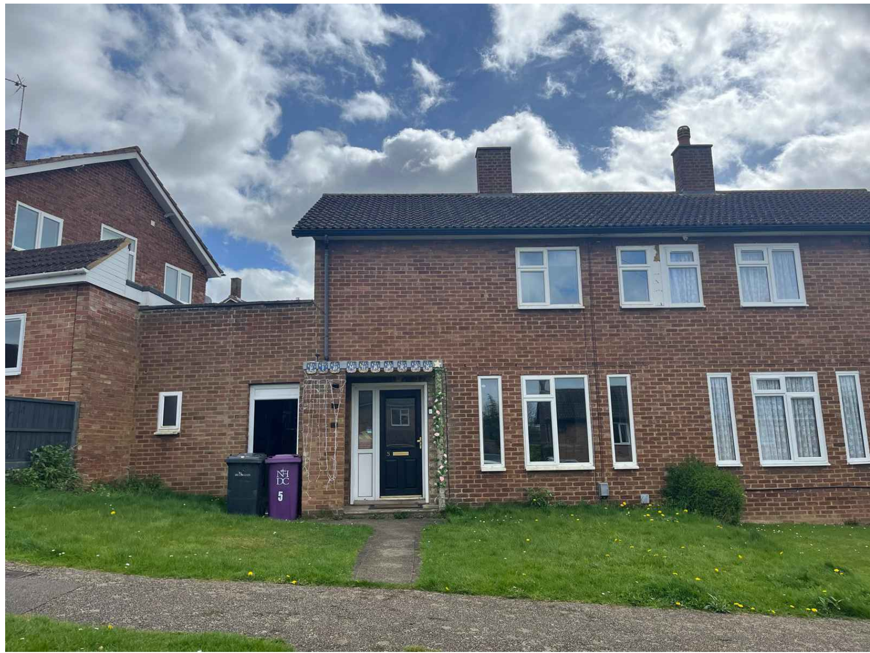
FRONT VIEW OF EXISTING PROPERTY
