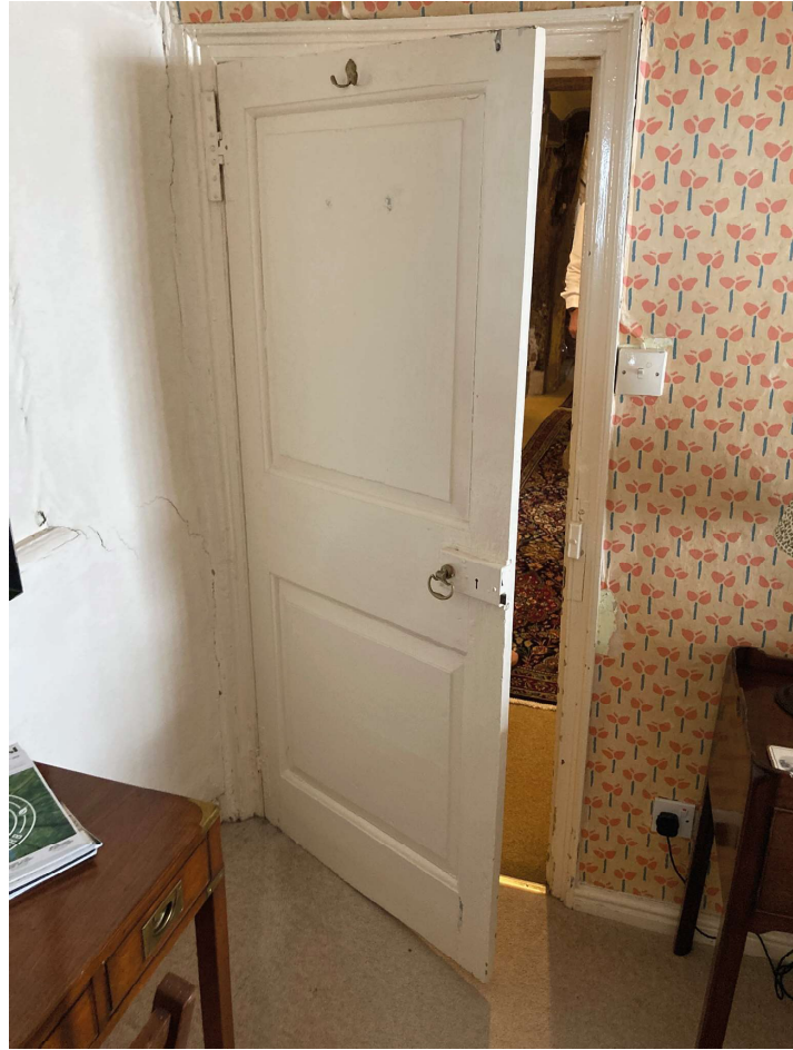
Photo of existing door, view from inside Bedroom 6
