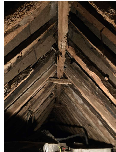
Photo of loft space over bedroom 5 looking south into the void over the ceiling above Bedroom 4 (15th Century Medieval Hall House)
