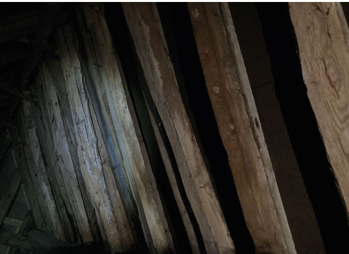
Photo 2025 showing historic rafters with modern rafters overlaid, likely done when the house was re-roofed in the 1980's. (Loft space of east west range of house).
