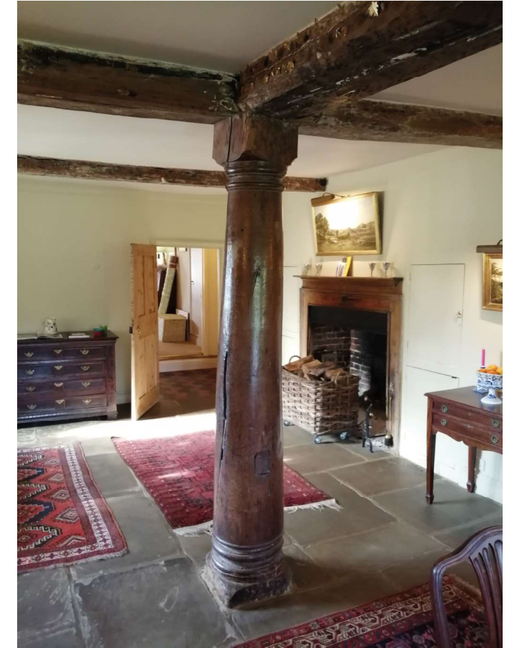
Photo looking at the ground floor area of the 15th Century Medieval Hall with the later extension east, removal of the wall and insertion of the round column in place of the wall. Fireplace is a 17th/18th Century addition, referred to as the north fireplace in the extracts from the Jon Lowe Heritage Report.
