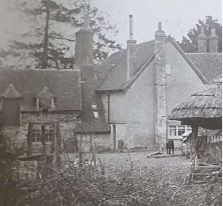
Photo 1908 facing the west end of the east-west gable range, chimney on the face of the gable no longer exists, GF window is now bigger and central. The render/brick exposed has changed over time.
