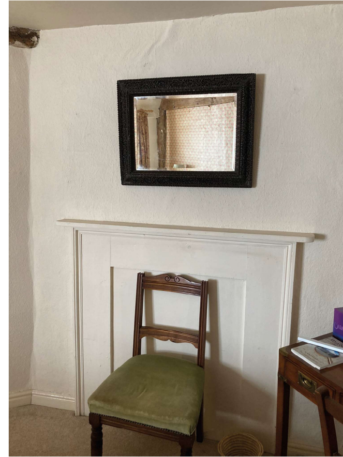
Photo of the 20th C chimney breast diagonally across the corner of Bedroom 6 with modern surround and blocked up opening. (North east corner of the gabled range).
