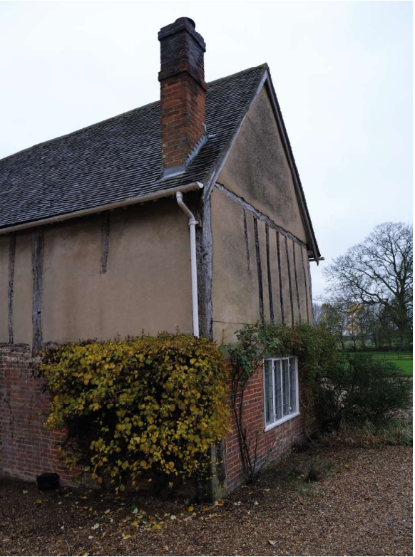
Photo 2020 north-west end of the east-west gable range (prior to conservation repairs of external fabric) showing changes since the 1908 photos.
