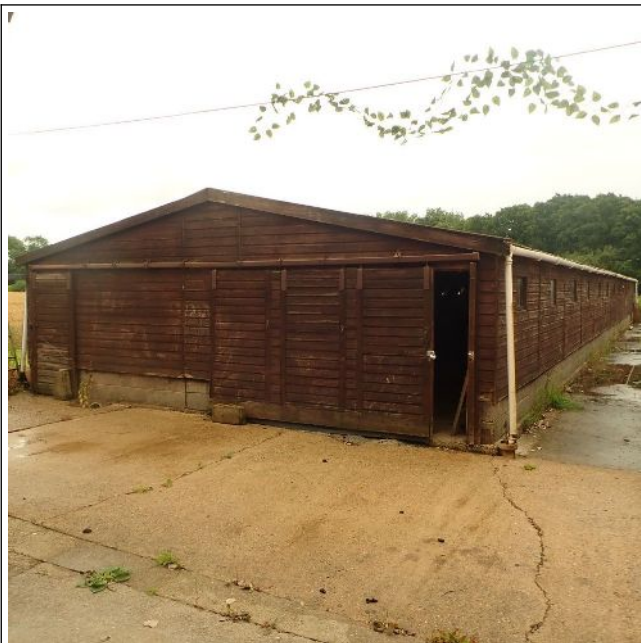
Figure 13: Building 3 - western end
