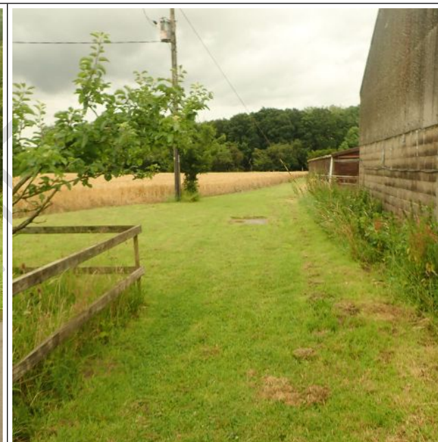
Figure 25: North side of main buildings with Philpott's Wood in distance
