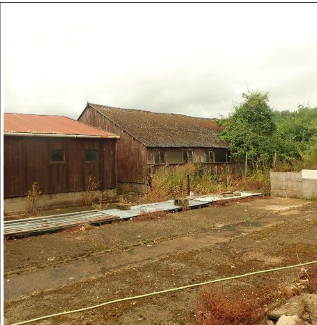
Figure 17: Building 4 and Building 5 from south side
