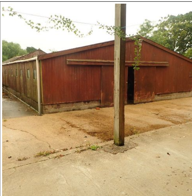
Figure 14: Building 4 - western gable
