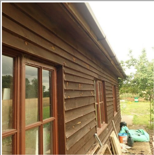
Figure 19: Building 6 - eastern wall looking north
