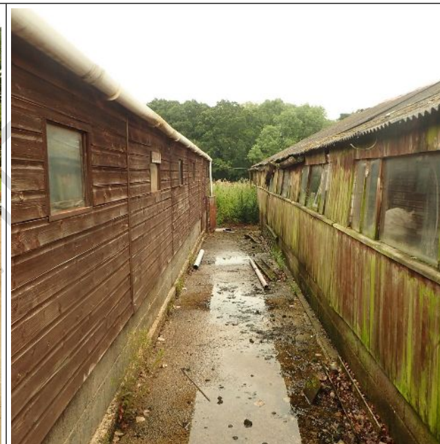
Figure 15: Building 2 to left with Building 5 to right
