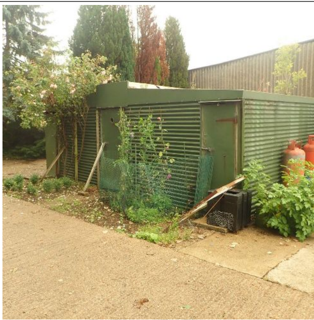
Figure 20: Building 7 from south side with Building 2 behind
