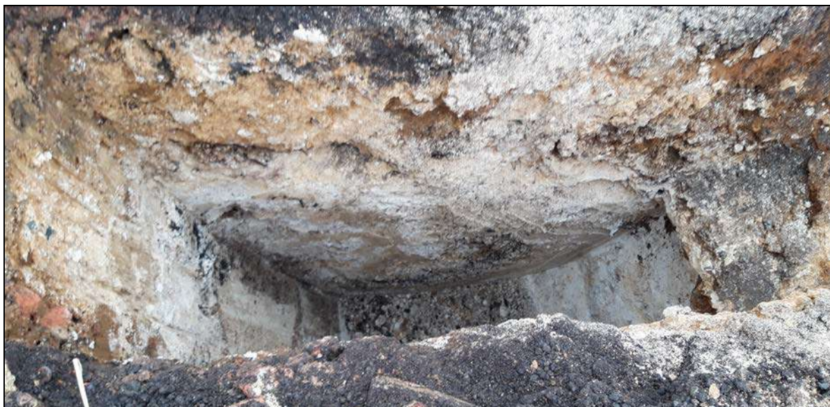
Photo 5 – TP2 base of pit.
