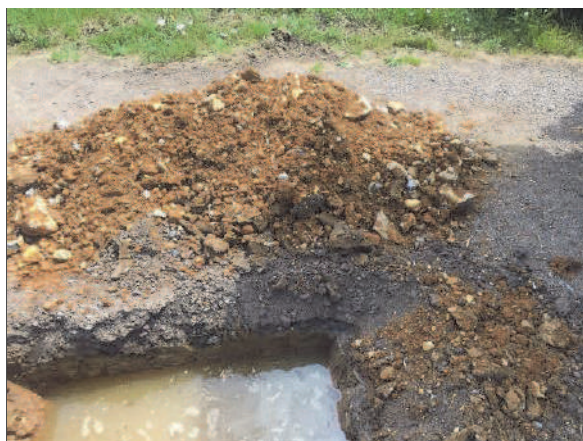
PHOTO 2 Trial Pit 3 (TP3)
