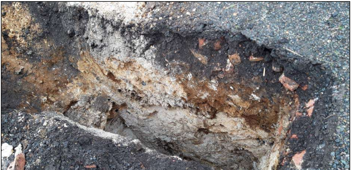
Photo 4 – TP2 top of pit.
