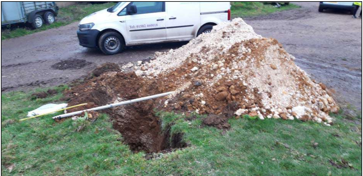
Photo 2 – TP1 location and spoil heap.
