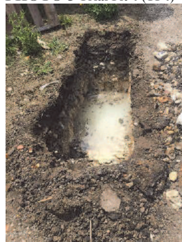
PHOTO 3 Trial Pit 4 (TP4)
