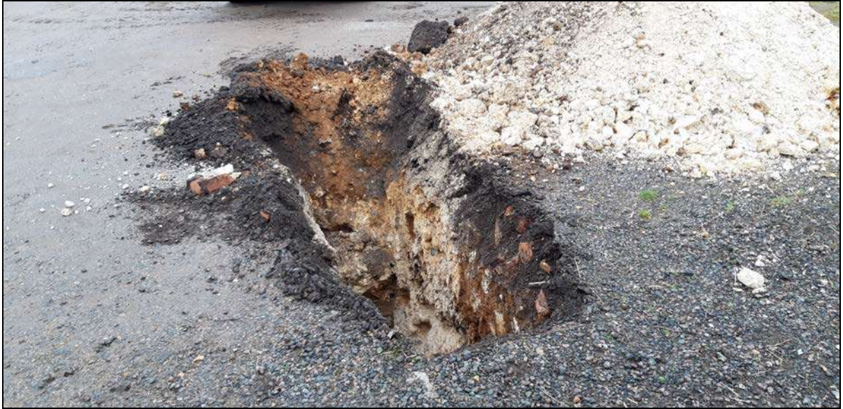
Photo 3 – TP2 location and spoil heap.
