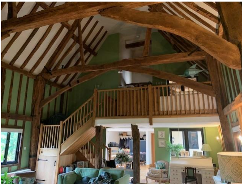
Interior of Belfry Barn looking east, showing existing staircase
