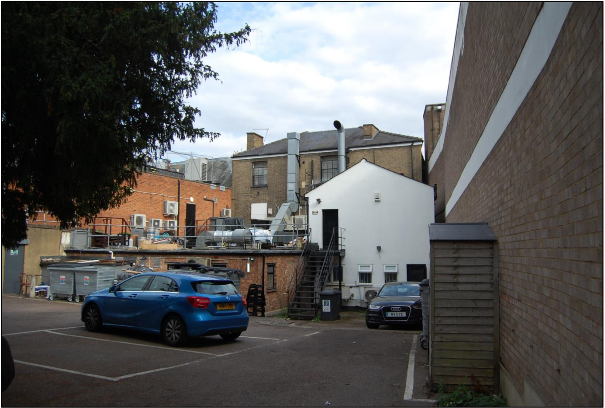
Existing rear car park
