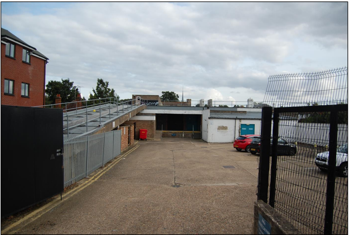
Existing rear car park and additional car parking accessed via vehicle ramp
