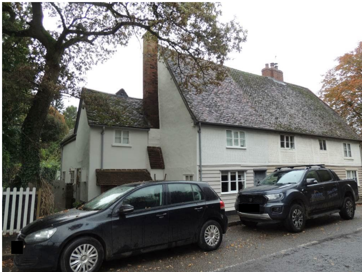
Photo 1: Front (eastern) elevation
