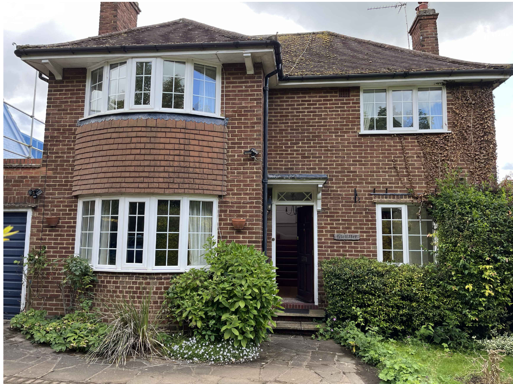
FRONT VIEW OF EXISTING PROPERTY
