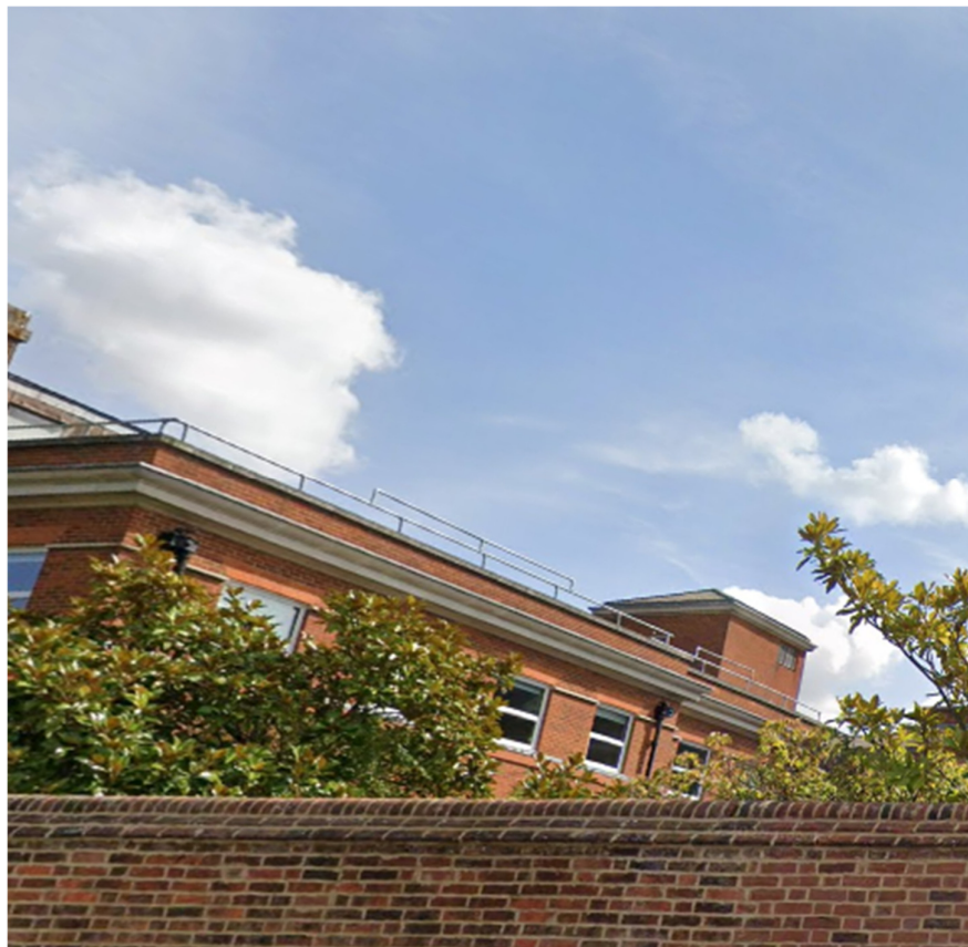
Photo 1: fall protection system at roof level of neighbouring Radcliffe House
