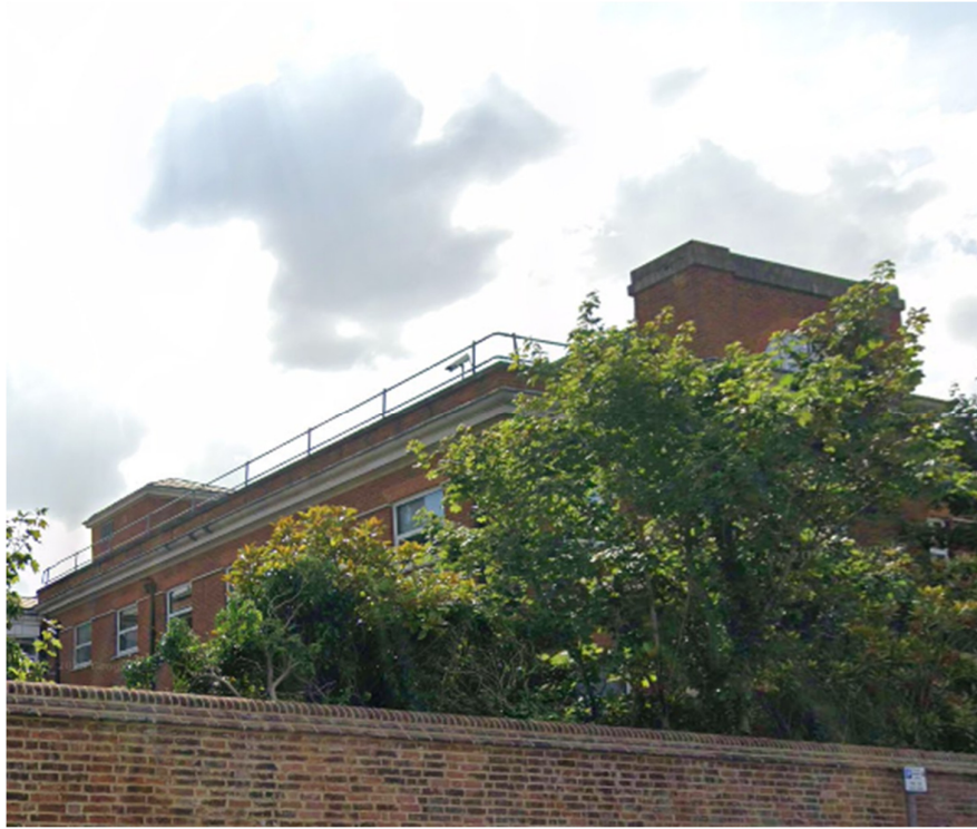
Photo 2: fall protection system at roof level of neighbouring Radcliffe House
