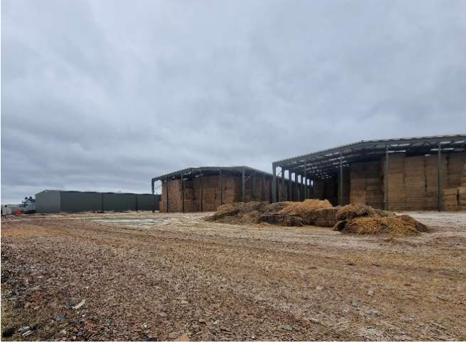
Photo 7: Existing off-site storage buildings.
