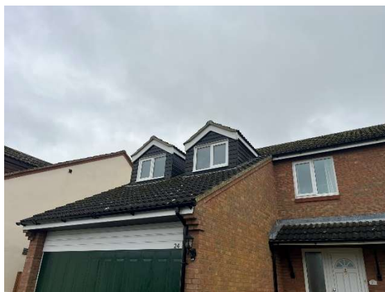
Photograph 6. Showing the intact dormer windows including the lead flashing and borage board. Showing the slightly lifting soffit.
