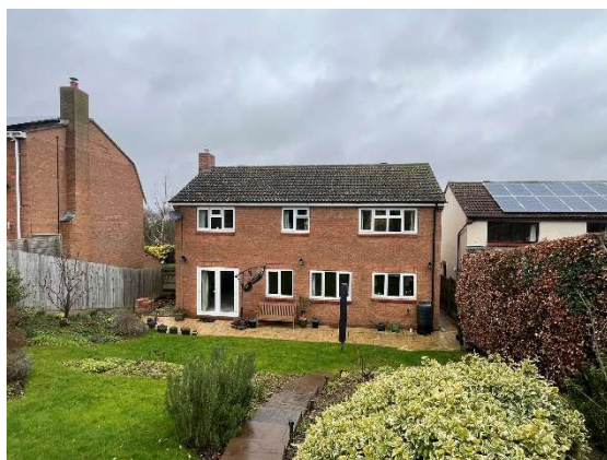
Photograph 2. Southern elevation of B1.
