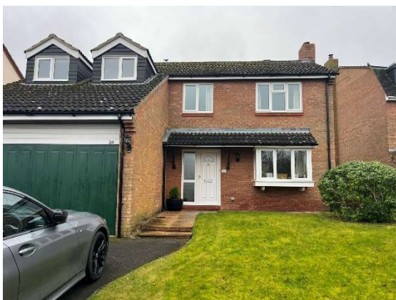
Photograph 1. Northern elevation of B1.
