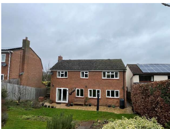
Photograph 11. Southern elevation of B1 and vegetated garden.
