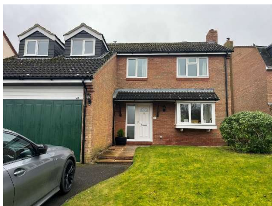
Photograph 10. Northern elevation of B1.
