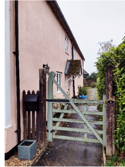
05 Entrance to no. 5 & north/side elevation from Westbury Farm Close.
