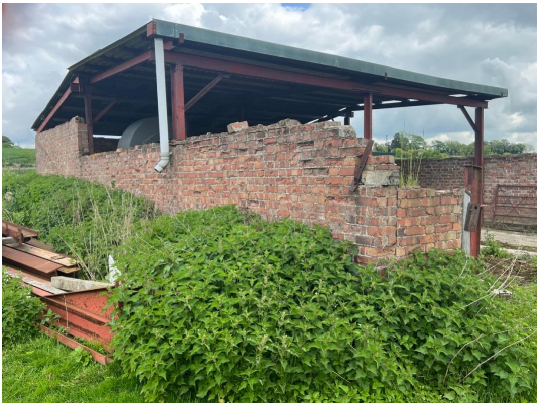
Figure 3-8 B4- open pole barn
