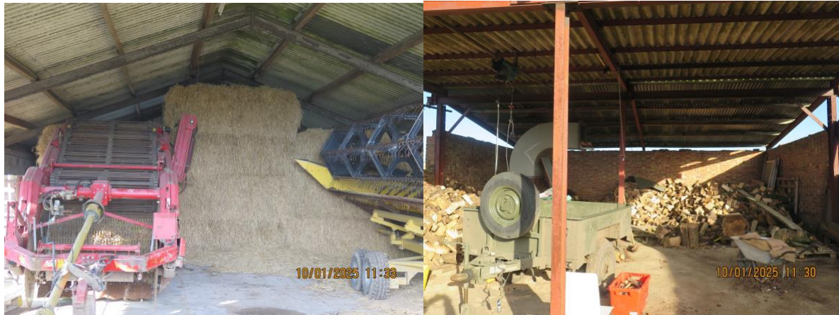
Figure 2 area at front of cattle shed and open sided pole barn
