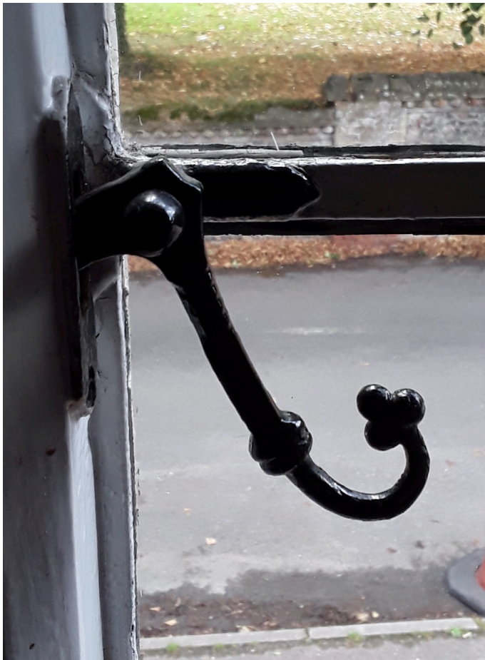
Photograph of Monkeytail Window Fastener scale nts
