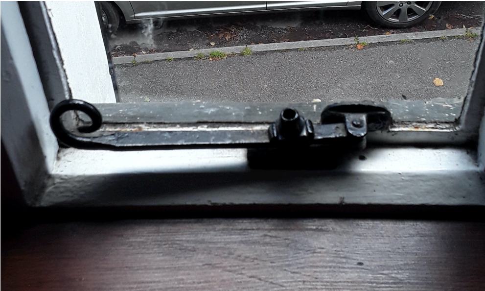
Photograph of Monkeytail Window Stay scale nts
