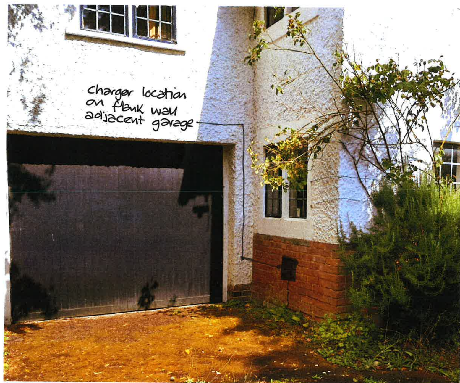
CHARGER LOCATION - FLANK WALL ADJ GARAGE.
