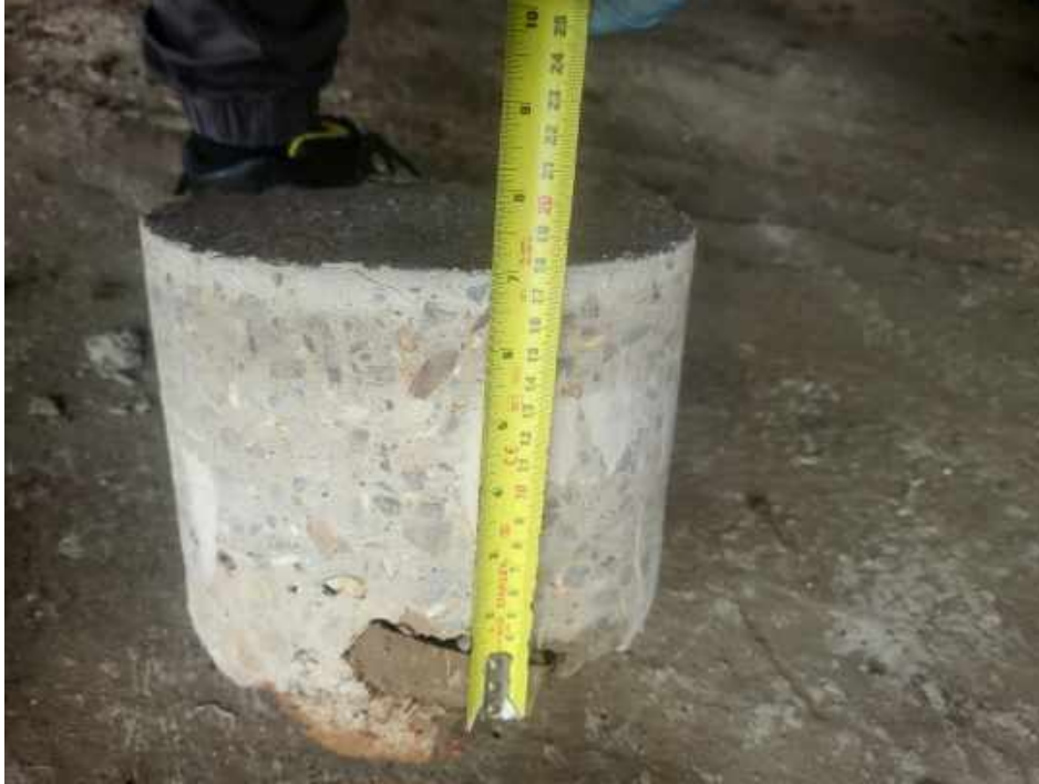
Photo 5 – Concrete Core from inside the barn (BH1)
