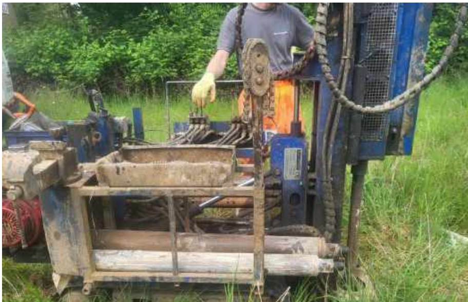
Photo 4 – Window sampling rig operating at BH2
