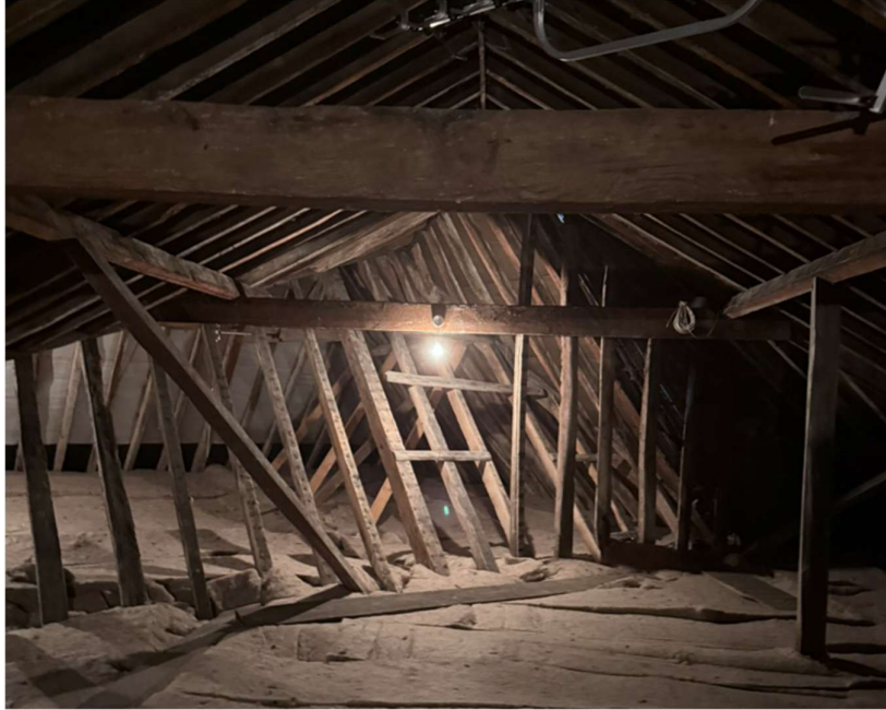
Fig.17 C17 range to Market Hill, with principal rafter truss with collar, tie, re-used flatways rafters and evidence of former location of battens on outer face of rafters
