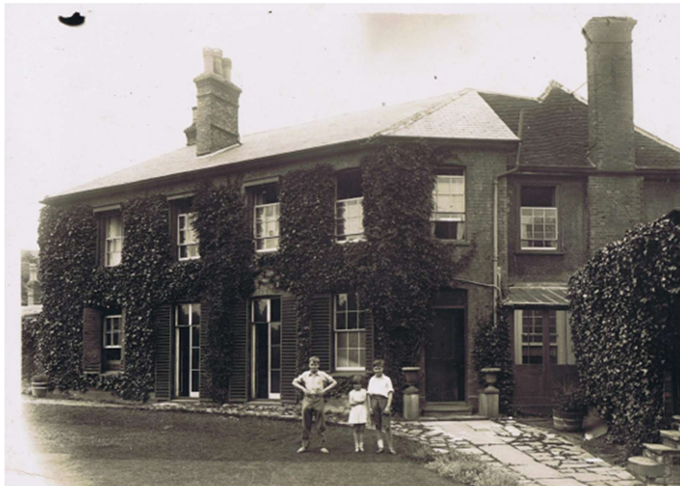
Fig. 3 Photo of Greenlawns c. 1930s with Dick Neale, June Etheridge and Nigel Etheridge. Note the brick garden front was not rendered at this time; the early part to R. has a tiled hipped roof and the C19, 5-window range, a canted lower pitch slate roof
