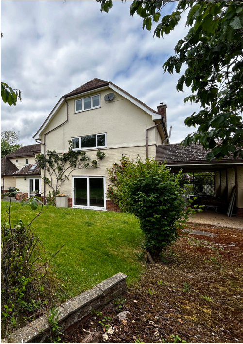
Rear elevation - hipped gable end and carport
