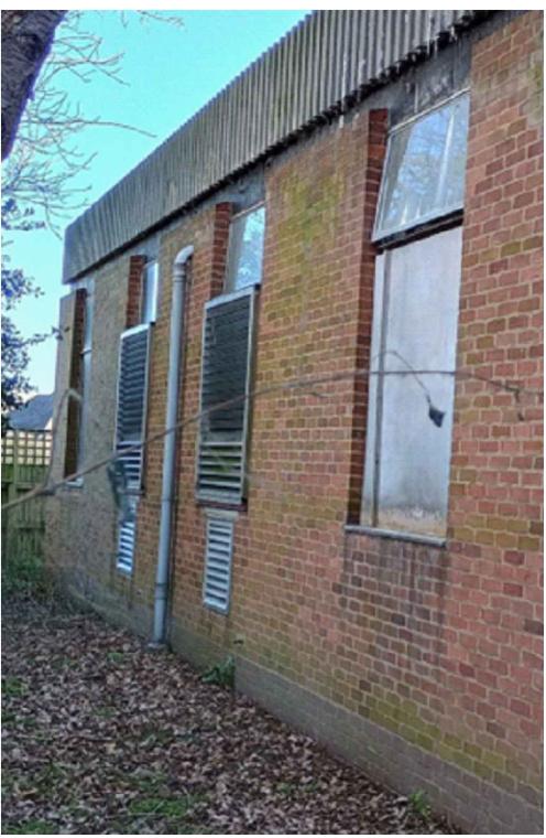
EXISTING LOUVRES ON WEST ELEVATION
