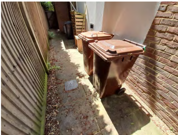
Side Walkway Fence with 20 Blackmore Way to left
