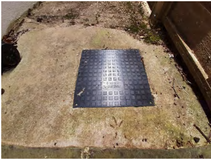
Side Walkway Drainage
