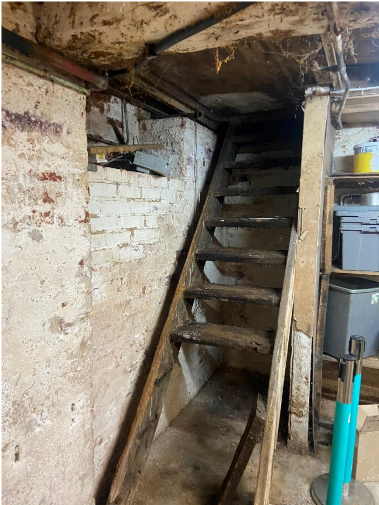
Photo of existing stairs to be replaced.
