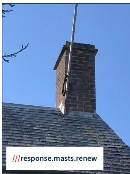
Figure 30. Slipped tiles around chimneys, providing crevices.
