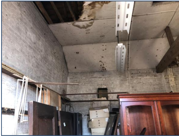
Figure 35a and b. The old stable's deteriorated ceiling.
