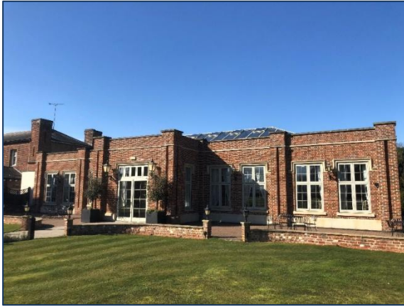
Figure 33. The Ballroom, east aspect.
