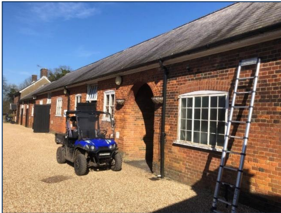
Figure 15. The old stables and boiler room.
