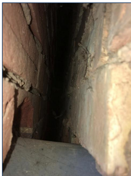
Figure 24. Cavity wall of cottage
