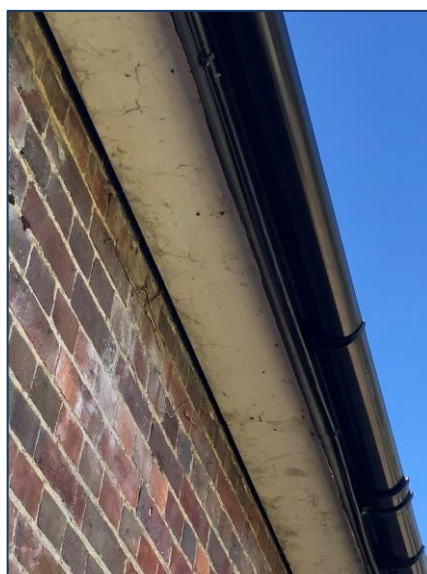
Figure 10. Gap in soffit on the east side of the old stable and boiler room stretching 13m (to ///risk.poetry.validated ) with a width of 1-3.5cm.
