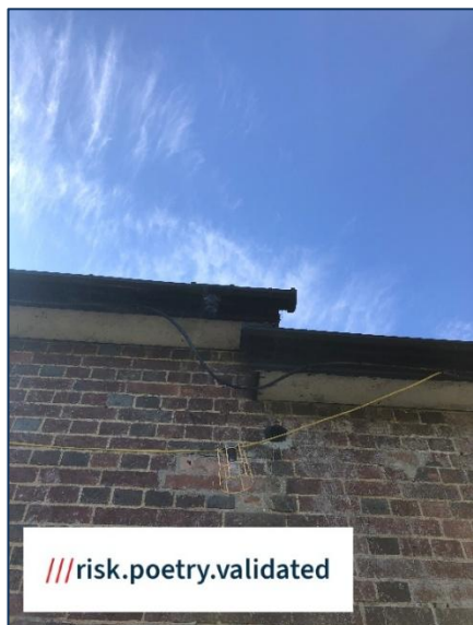
Figure 11. Intersection between the two soffits
