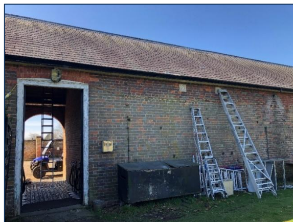
Figure 8. The alleyway running between the boiler room and old stable, containing the open loft hatch.
