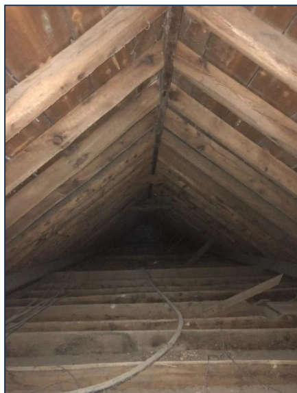
Figure 2. The loft void within the old stable and boiler room.
