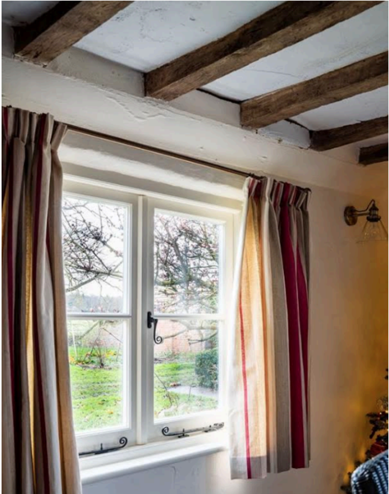
IMAGE 2: Interior of timber-framed casement window with 8.15mm vacuum insulated glass (VIG) and putty glazing. Note period appropriate handle and stays.
