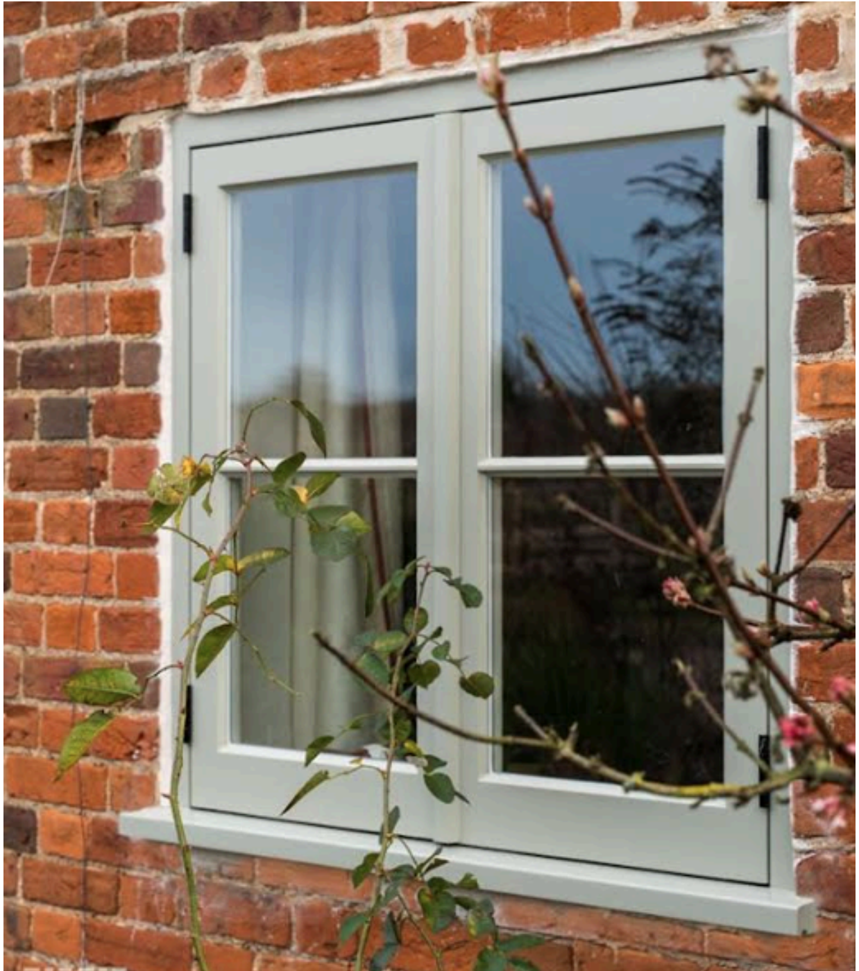
IMAGE 1: Exterior of timber-framed casement window with 8.15mm vacuum insulated glass (VIG) and putty glazing. Note that no glass cavity or rim is evident as with standard double-glazing.
