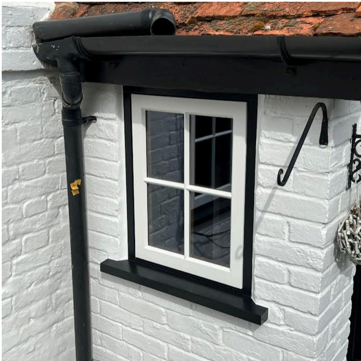
IMAGE 4: Exterior of Georgian-paned timber-framed casement window with 8.15mm vacuum insulated glass (VIG) and putty glazing.
