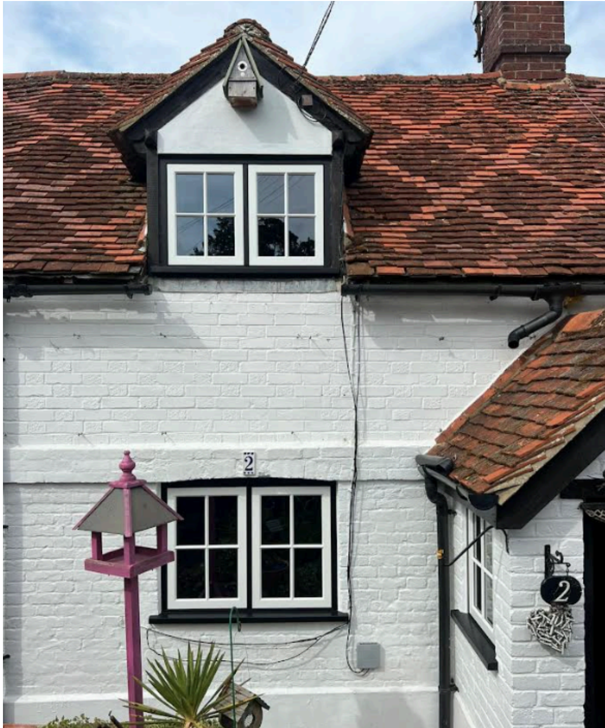
IMAGE 3: Exterior of Georgian-paned timber-framed casement windows with 8.15mm vacuum insulated glass (VIG) and putty glazing.
