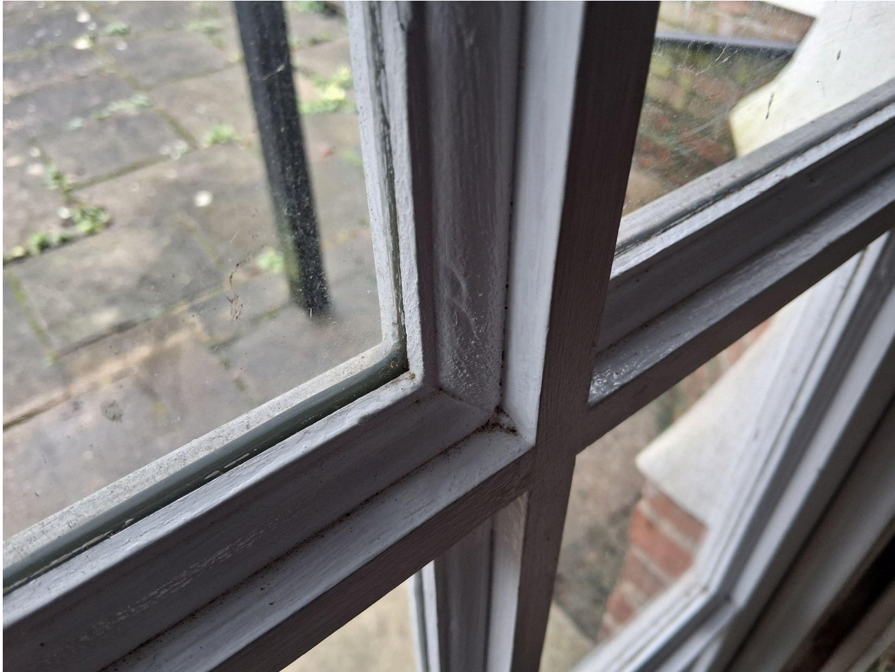
French doors 3: As these doors were replaced more recently than the windows, the style does not match any of the windows.
