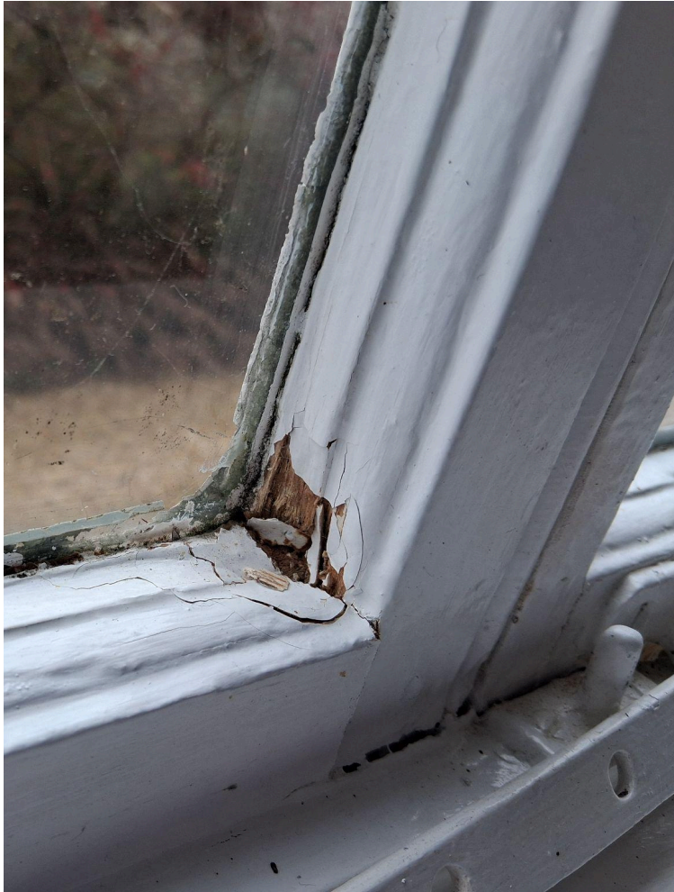
Window 8: Both inside and outside of the frame are heavily rotten and soft to the touch.
