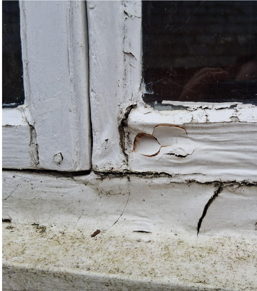
Window 8: Both inside and outside of the frame are heavily rotten and soft to the touch.
