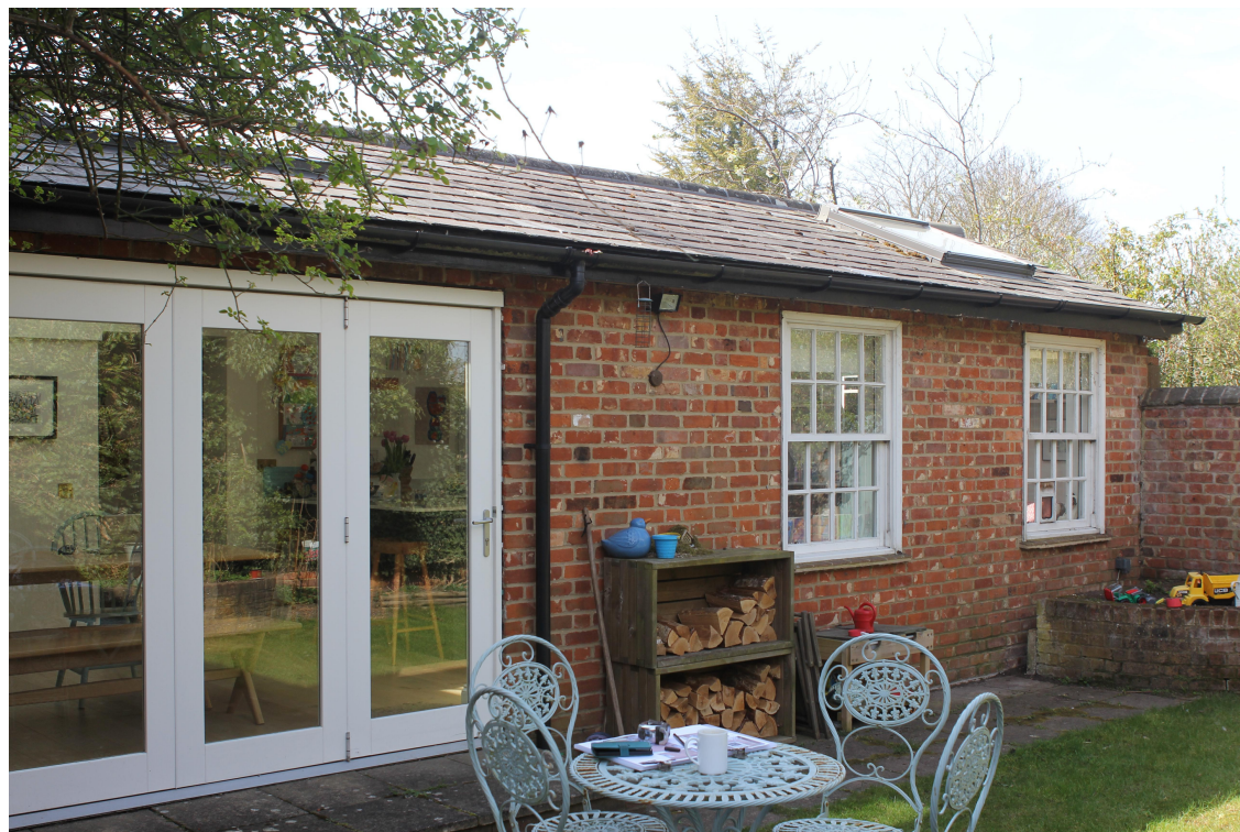
Ground floor rear extension
