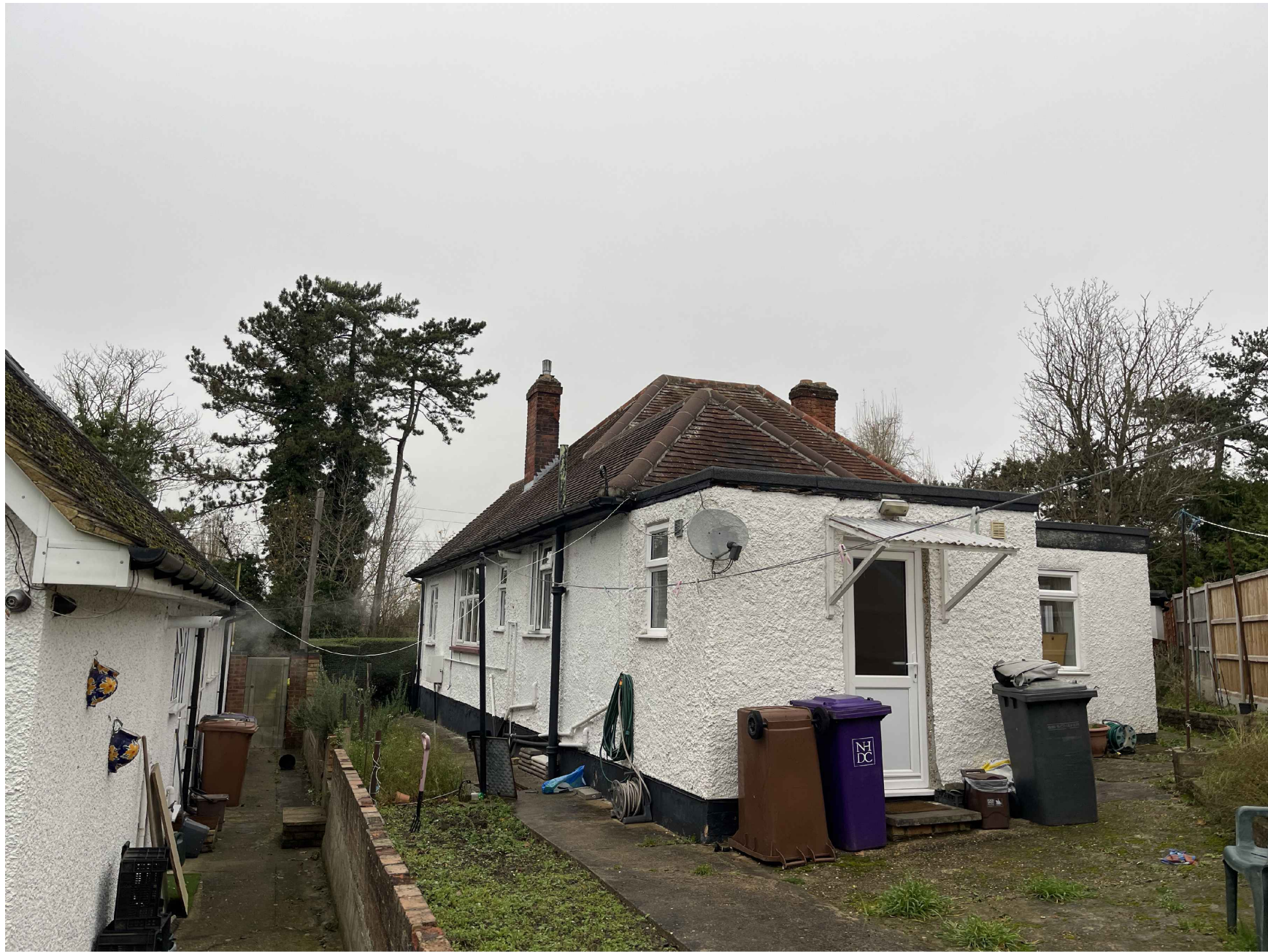
REAR / SIDE VIEW OF EXISTING PROPERTY
