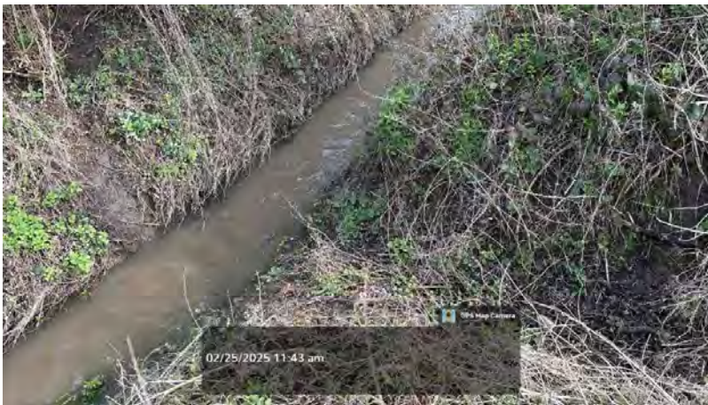
Photograph 3 Discharge of Unnamed Minor Ditch into the Cat Ditch along the northern site boundary
