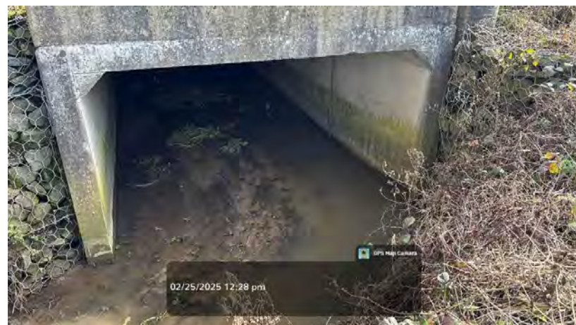
Photograph 6 View of downstream face of A1 culvert (other side of A1)
