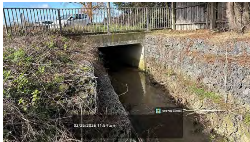
Photograph 5 View of upstream face of A1 culvert
