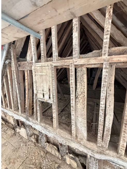
West End of North Wing, Upper Levels
