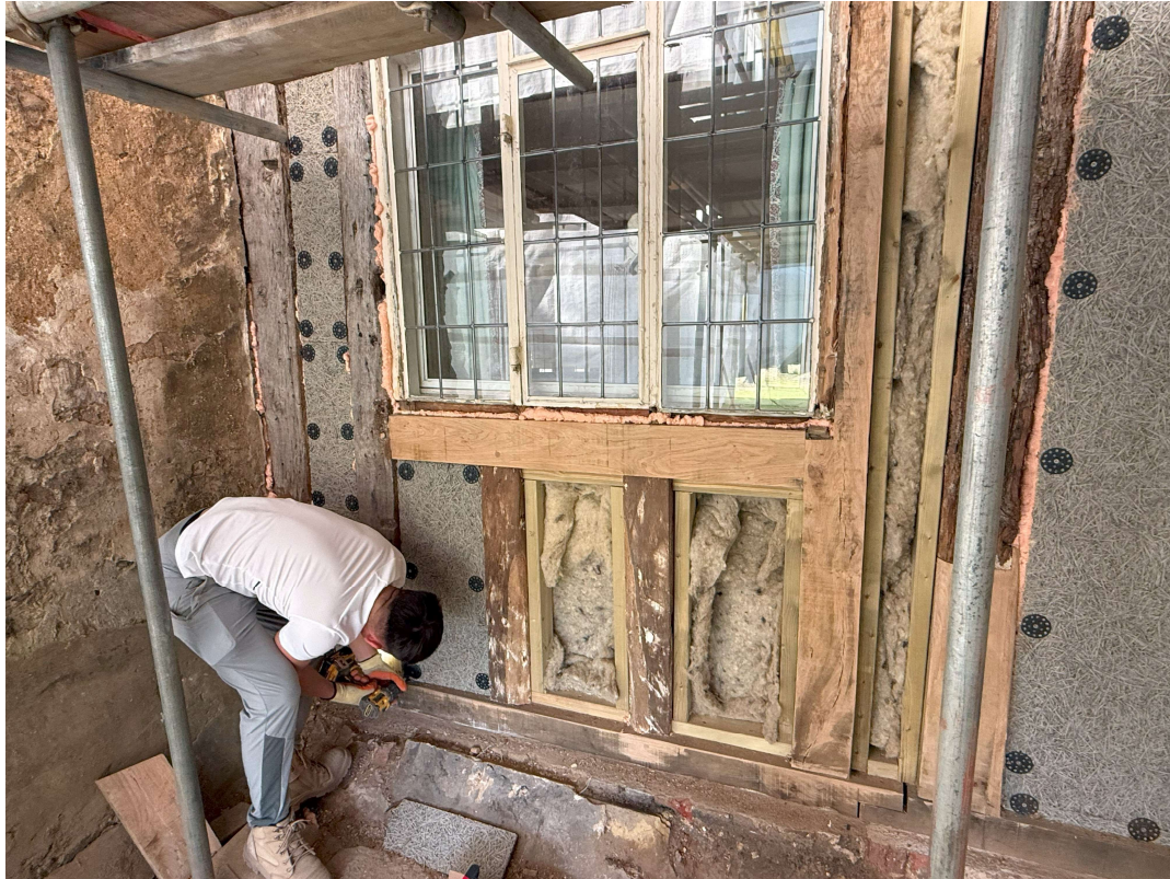
East Elevation of East Wing (between Chimney and Stair Well)
