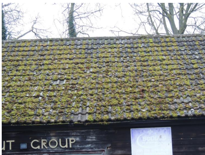
Photo 10: Note tight seal to roof tiles
