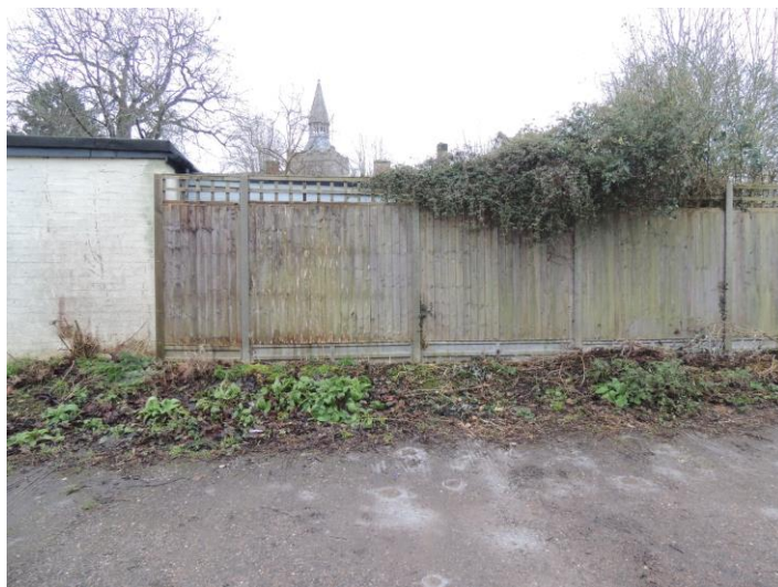
Photo 17: Southern boundary of the site
