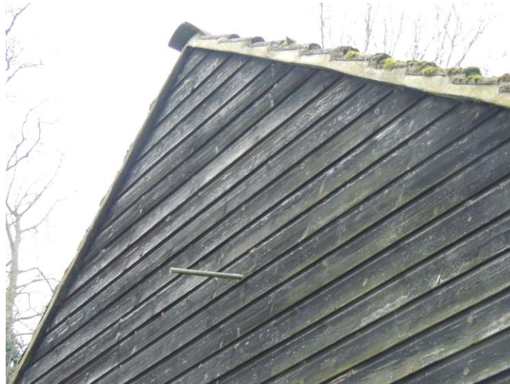
Photo 12: Note tight seal to gable and cladding
