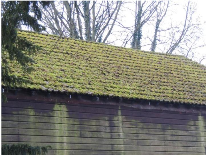
Photo 11: Note tight seal to roof tiles and cladding
