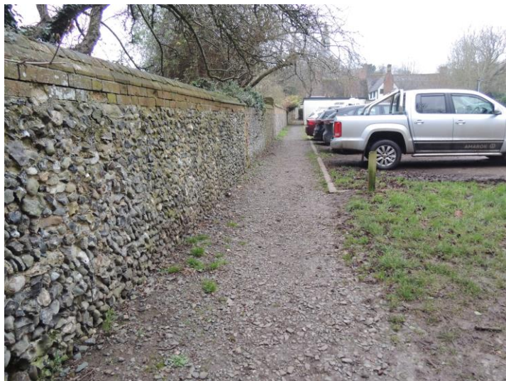
Photo 16: Looking southwards along walled eastern boundary. Note lack of habitat for reptiles
