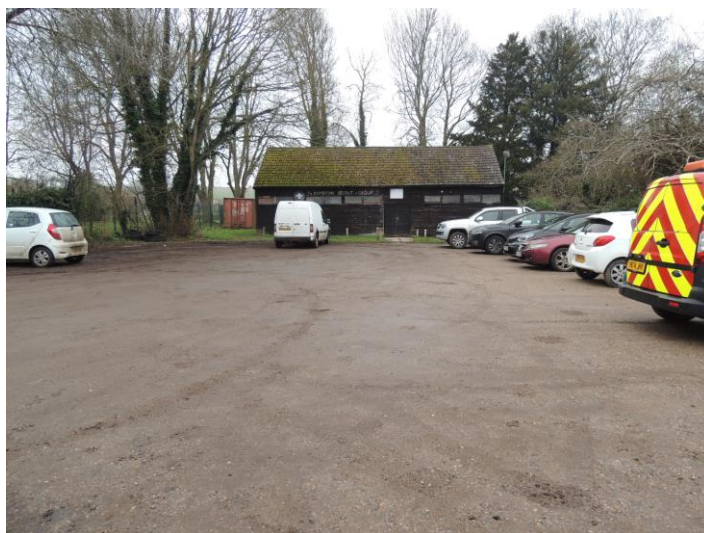
Photo 18: Looking northwards at the site
