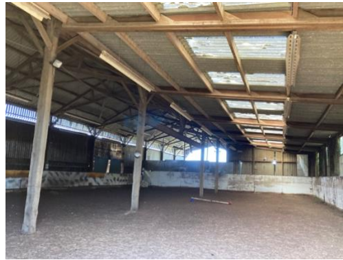
Photograph 14: Internal of Building B2
