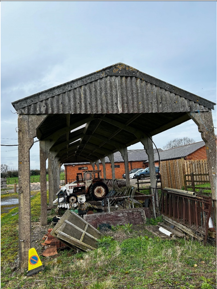
Photograph 4: Building 2 in the north of the site.
