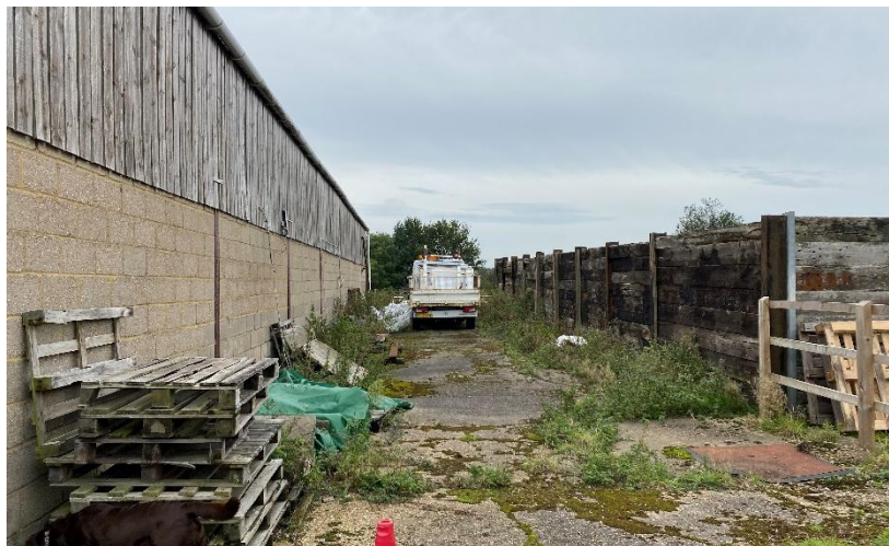
Photograph 4: View looking south showing (west side) elevation of agricultural building to be converted to business and storage use; open storage yard right of picture (behind timber sleepers) to be replaced and used for parking for the new business units.
