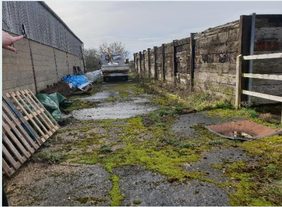
Hardstanding between barn and yard
