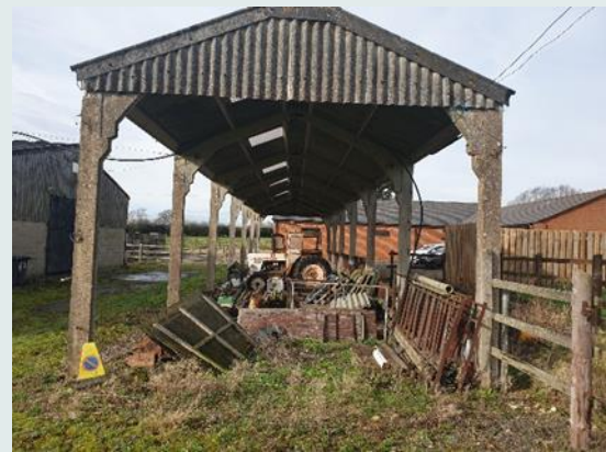
Open barn structure to north
