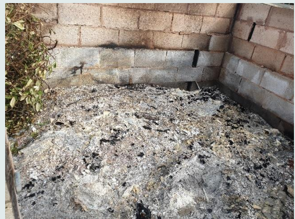
Burning pit within brick surround
