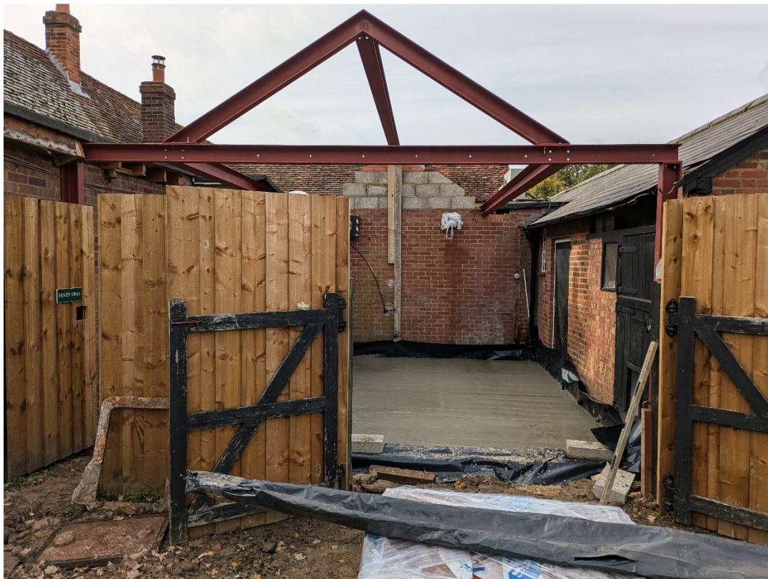
Courtyard under construction October 2024
