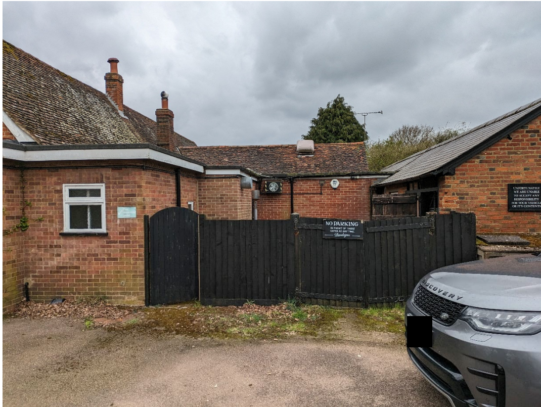
Courtyard prior to start March 2024
