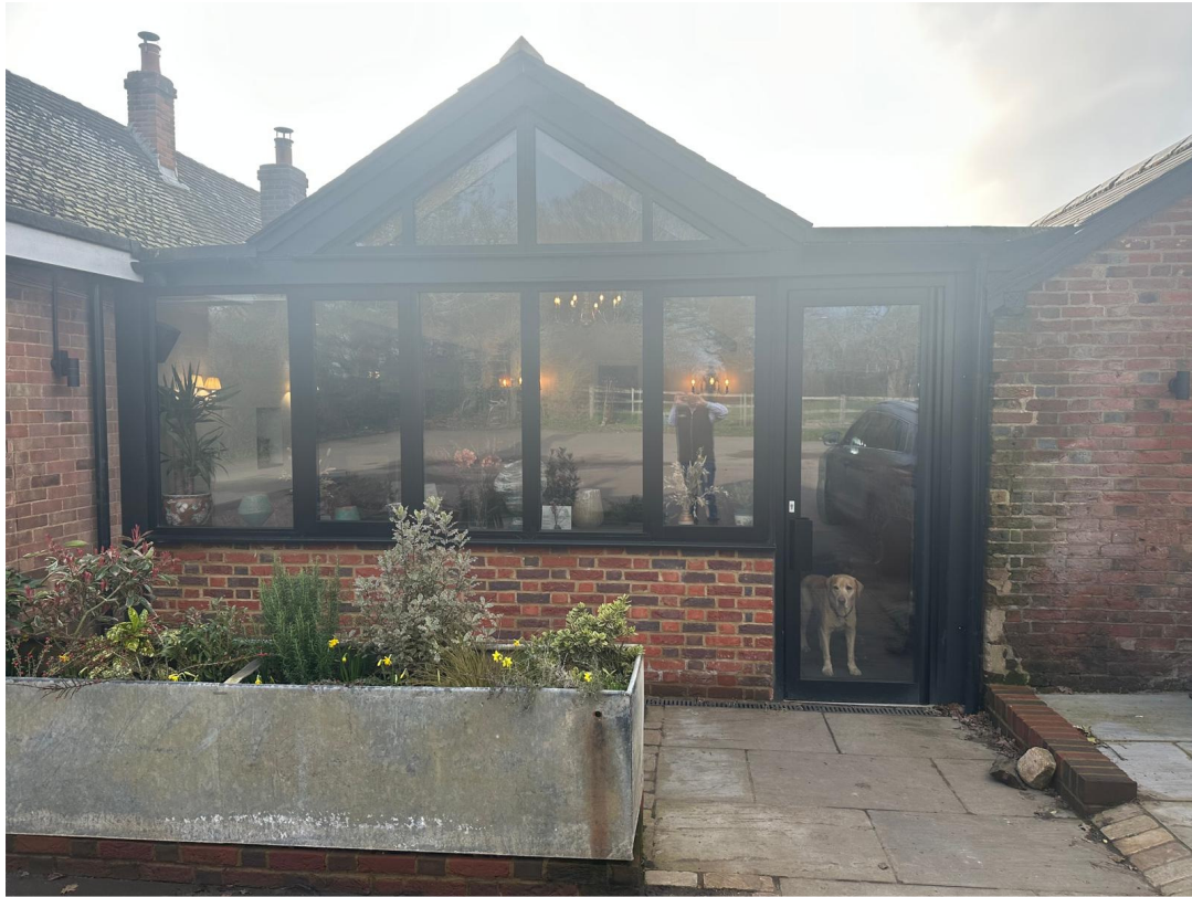
Courtyard completed March 2026
