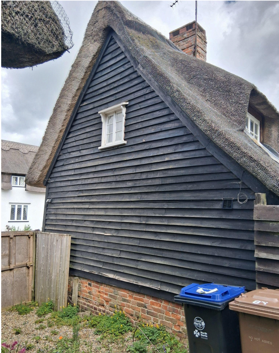
South_01: This window on the south side of the house is not being replaced.
