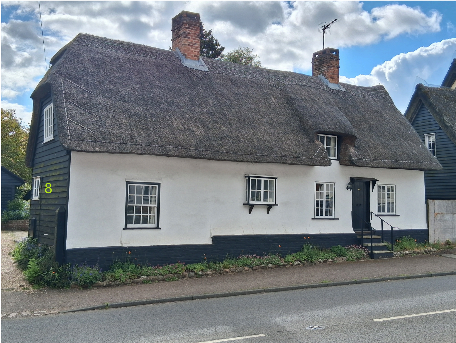
Front_01: Front of house and north side. None of the windows on the front of the house are to be replaced. Only the downstairs window (8) on the north side is to be replaced.
