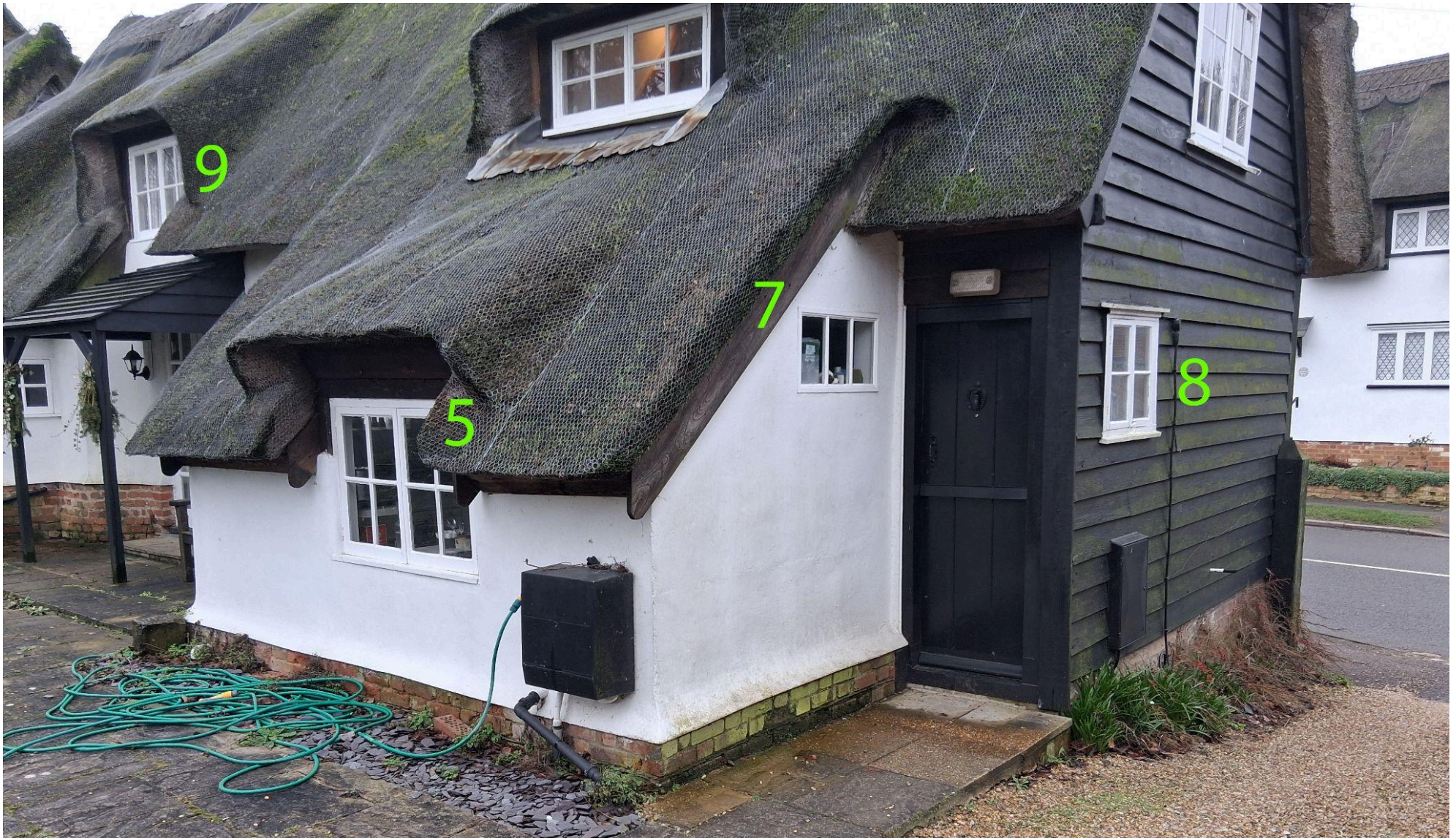
Rear_03: Kitchen (5 & 7), middle bedroom (9) and side of house (8) windows to be replaced.
