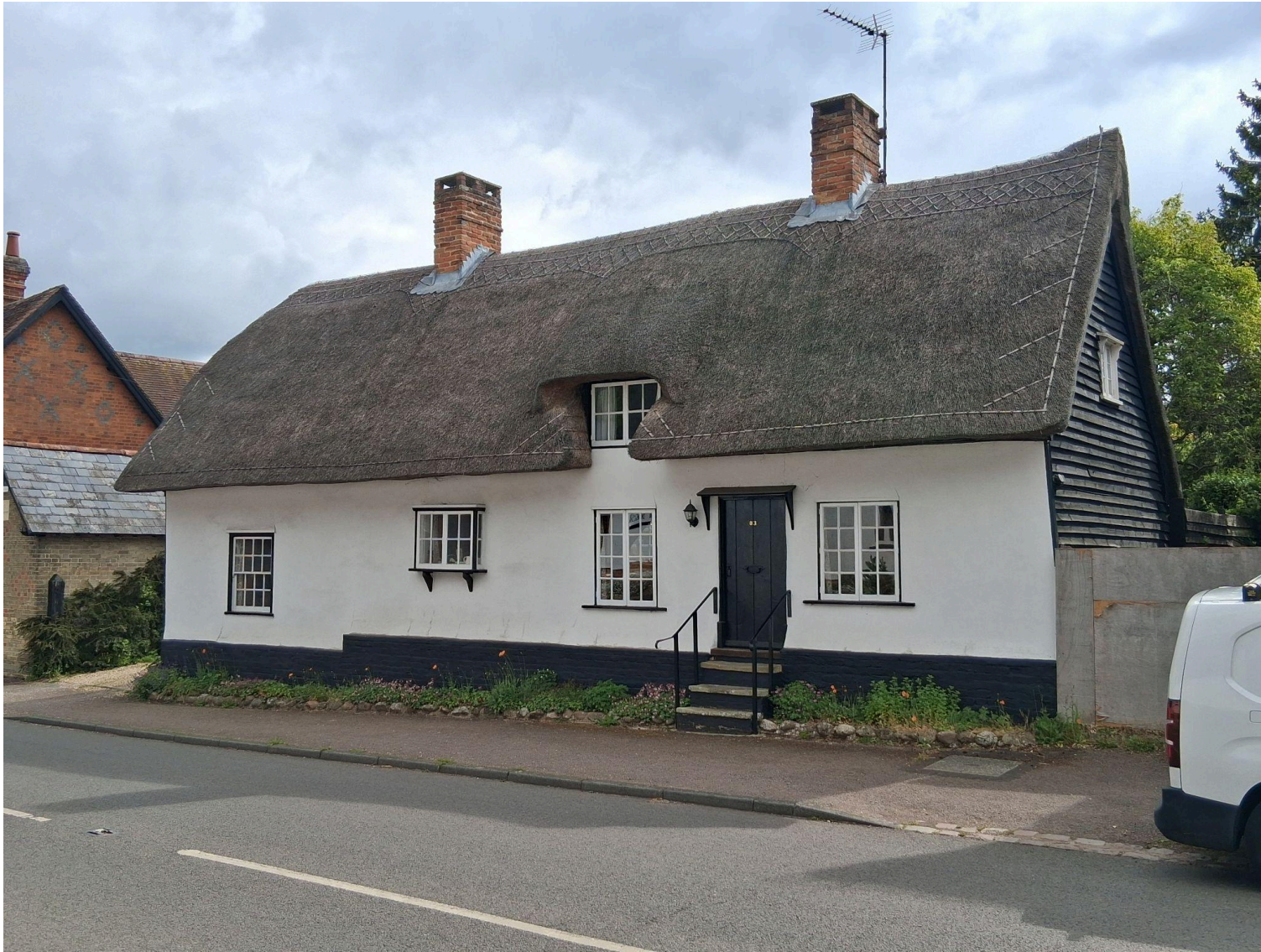
Front_02: None of these windows on the front or south end are to be replaced.
