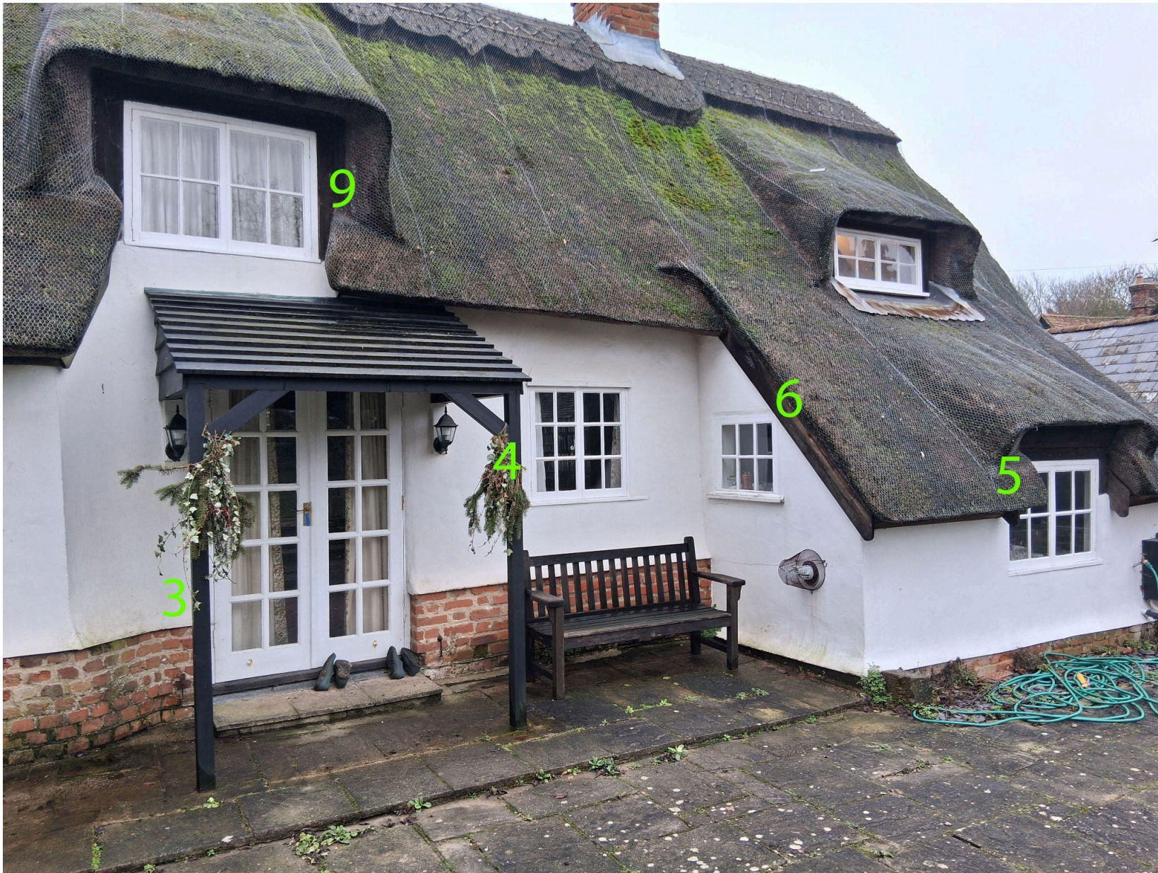
Rear_02: Living room (3 & 4), middle bedroom (9) and kitchen (5 & 6) windows to be replaced.
