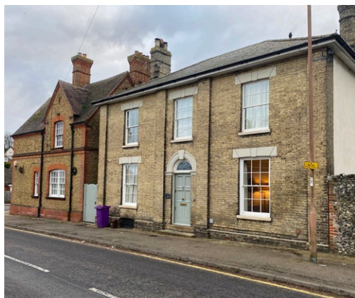
GEORGIAN BUILDING ON MARKET HILL
