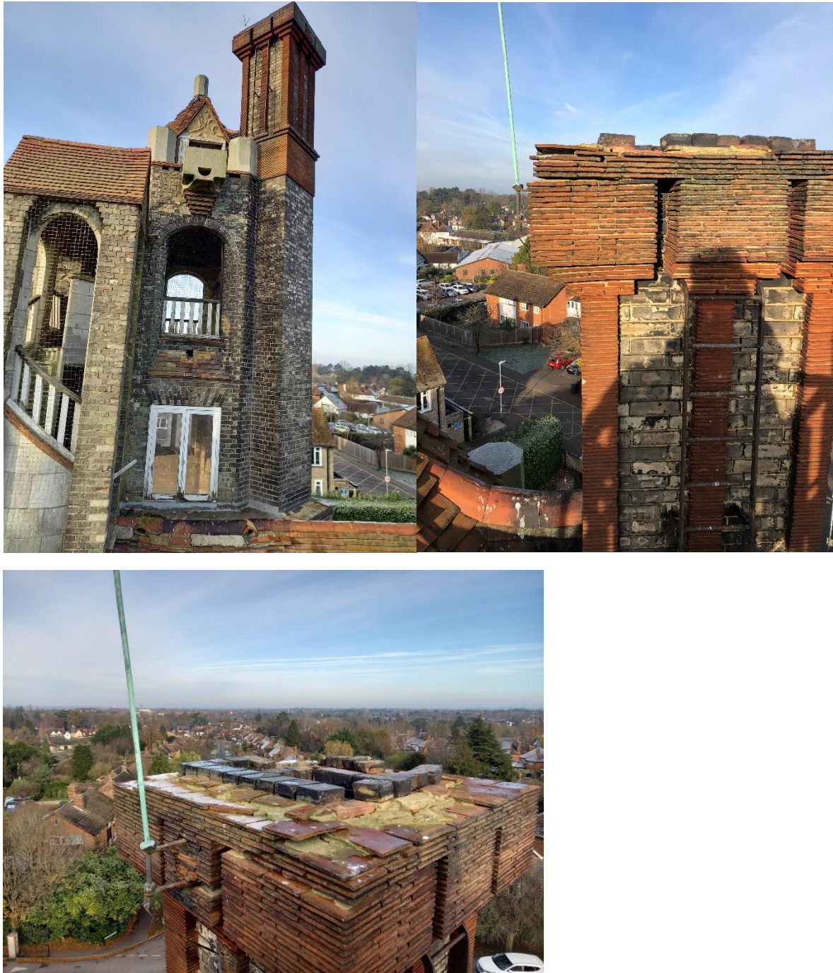
Close up photographs showing the current condition of the tile creased corbel
