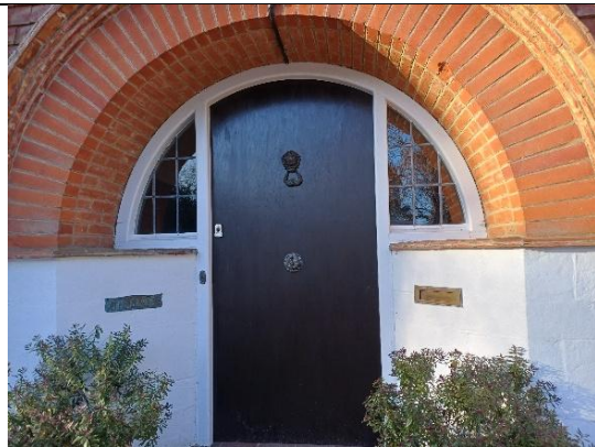
Entrance windows (retained)
