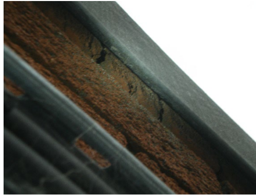
Feature 2: Over hanging lip of the roof. North east elevation
