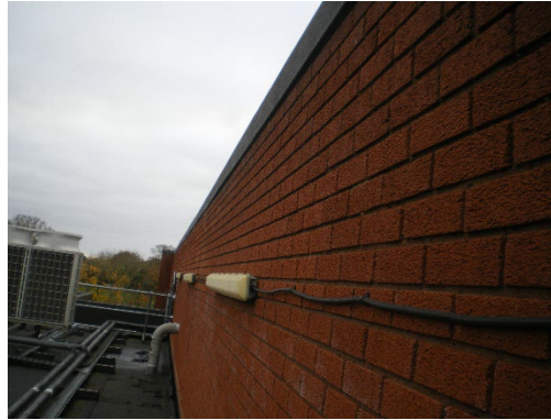
Feature 6,7 & 8 example: Long metal lips folded over the top of the wall from the roof on the northeastern and southeastern elevations.
