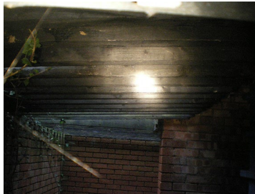
Feature 4: Roof in 2nd shed
