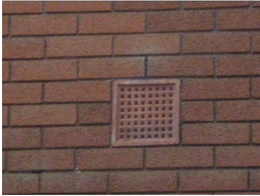
Feature 5: Weep holes above vent bricks
