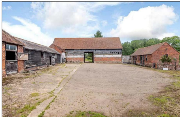
Plate 3: General view of barn and attached outbuildings at Rye End Farm looking N
