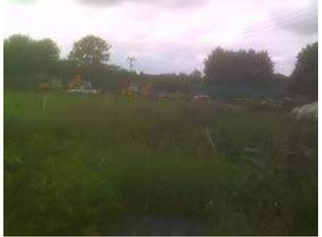
View looking north from location S
