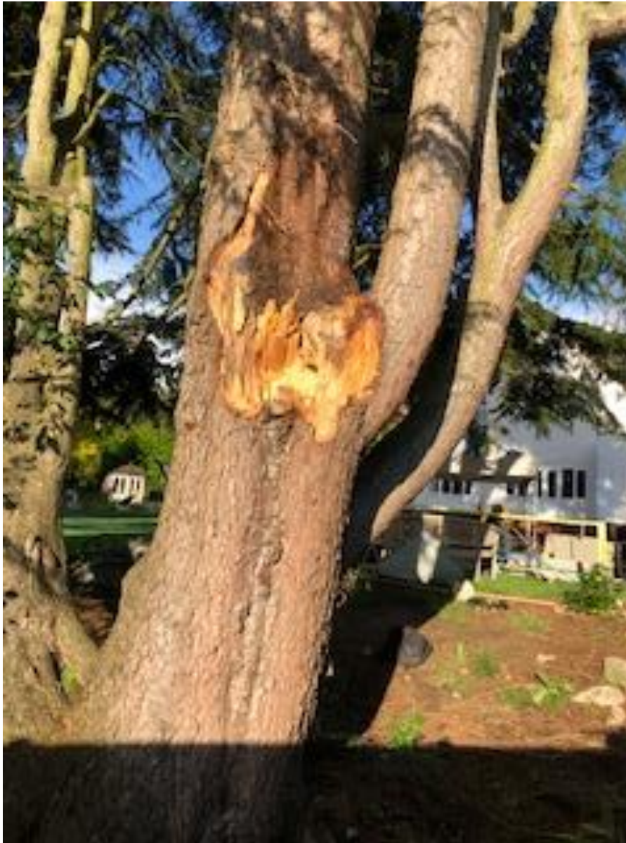
PHOTOGRAPH NO. 3 – BRANCH BREAKOUT POINT ON NORTHWESTERN SIDE
