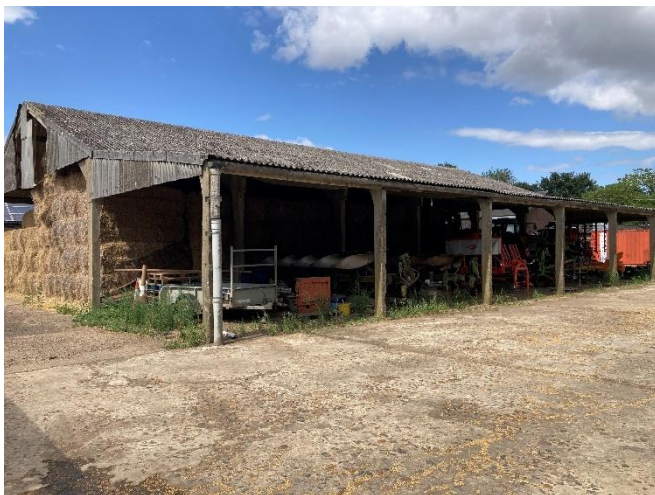
Barn 12 viewed from the south east.
