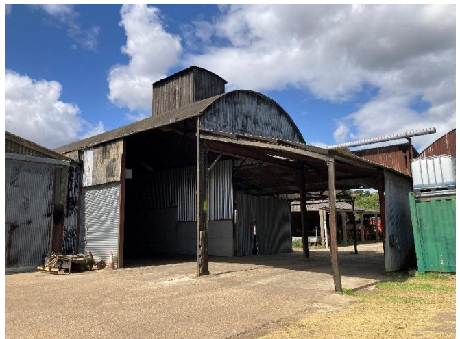
Barn 15 viewed from the south east, incorporating a rectangular roof structure.
