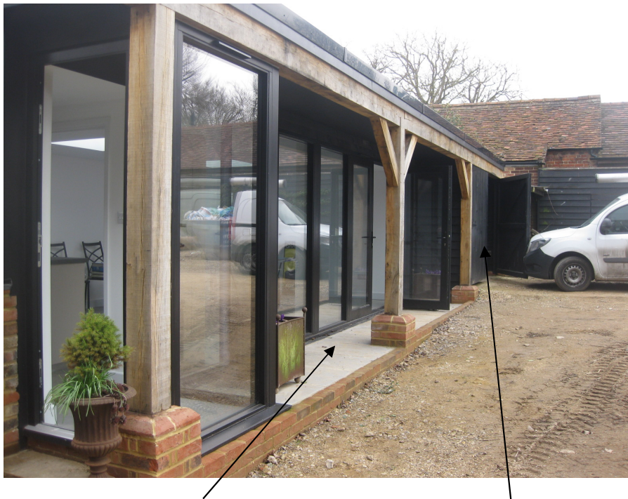
Existing office conversion in foreground
