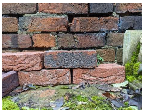
Olde Welwyn red multi bricks adjacent to the original brickwork
