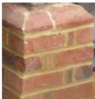
Olde Welwyn red multi bricks used for office conversion
