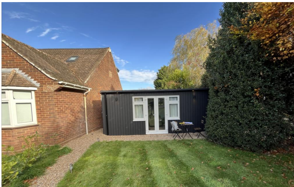
Figure 2 – Photograph of the existing outbuilding adjacent to main house
